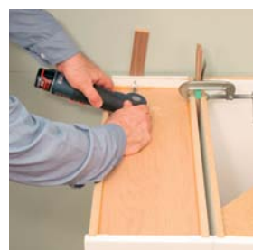
Installing Base Cabinets p. 167
