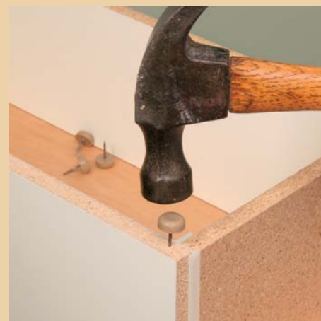
Tack glides are inexpensive flood insurance for base cabinets in moisture-prone areas.
