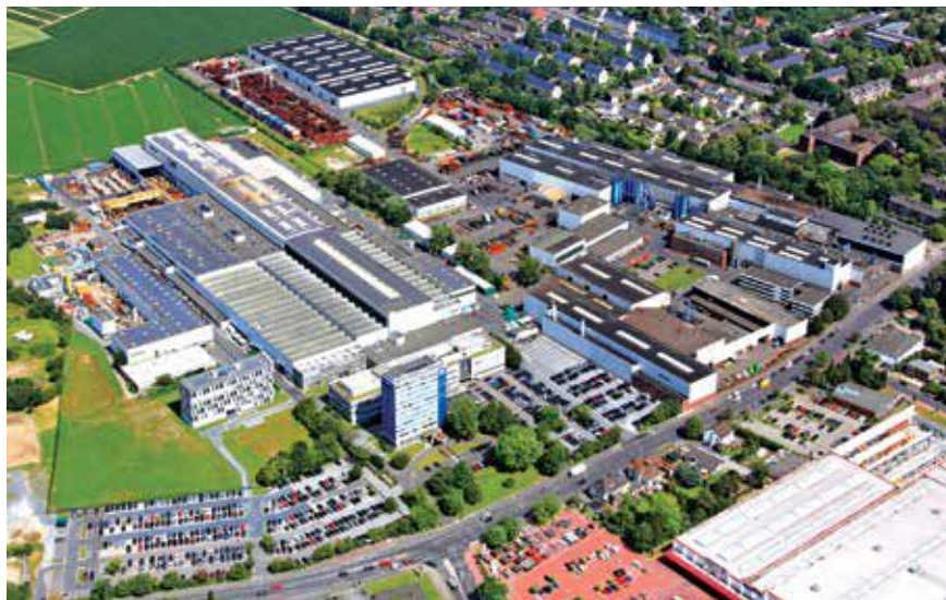
The production facilities of Siempelkamp's machine and plant building at Krefeld, Germany.
