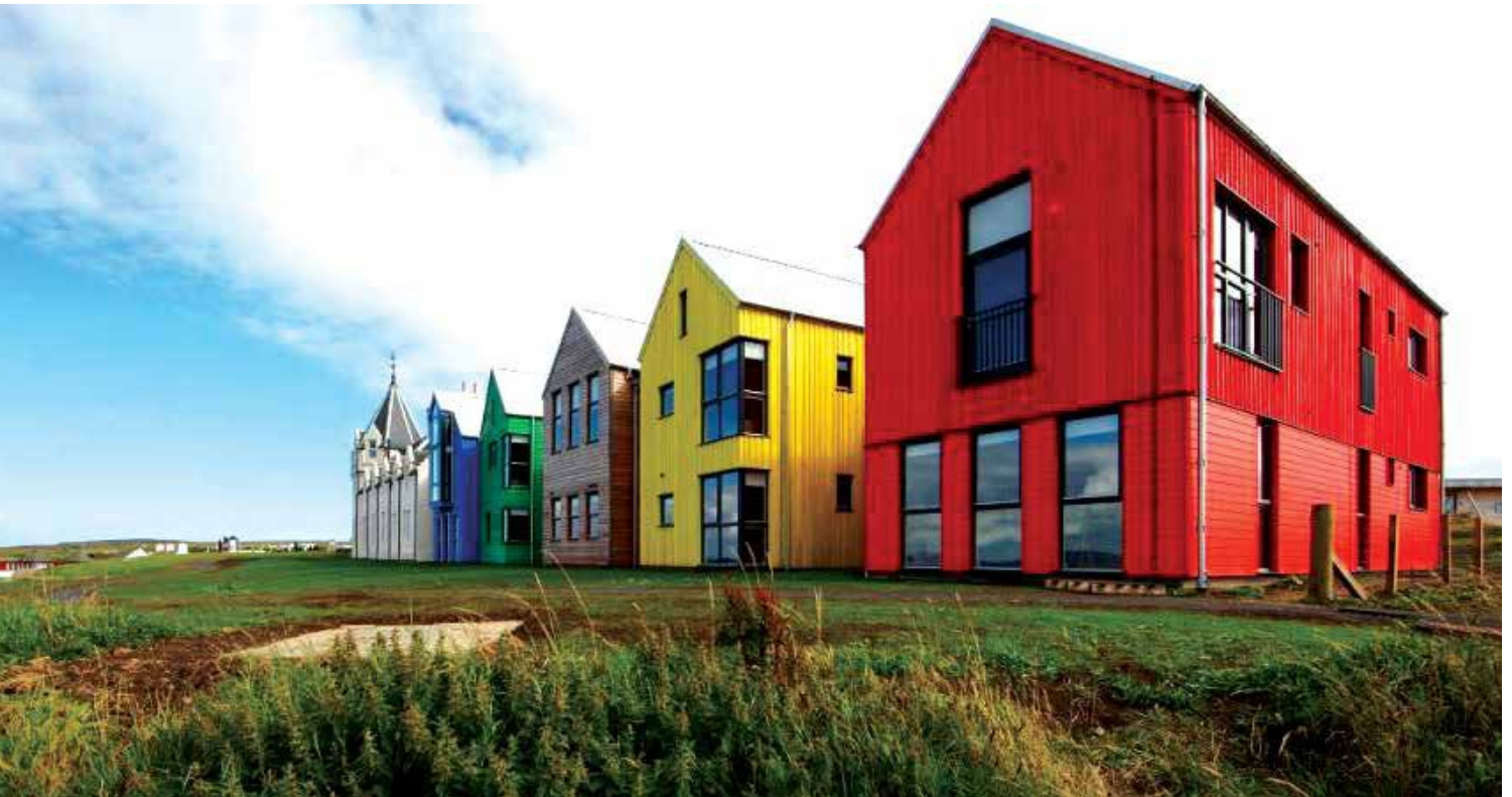
Vacuum-coated boards from Scotch Lark adorn this building in Northern UK.
