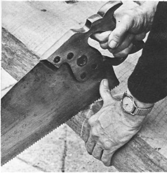
129 Cross-cutting plank with handsaw
