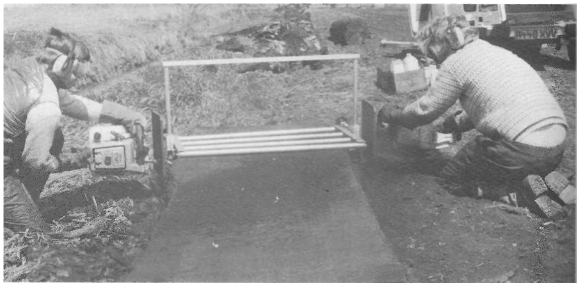
7 Subsequent cuts do not require the ladder support. (By courtesy of Philip Cole)
