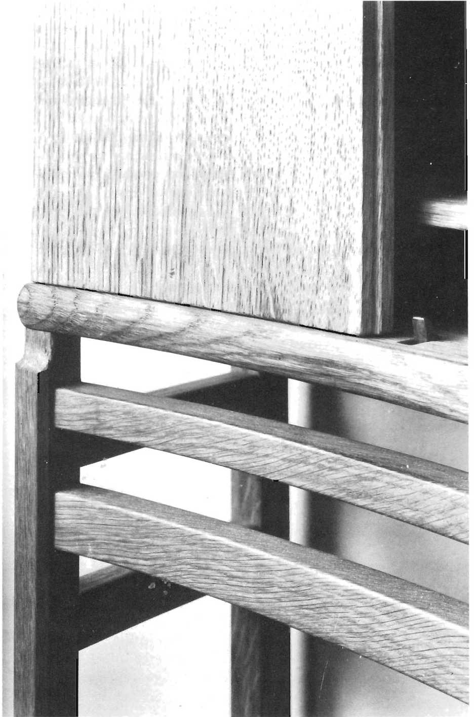
Oak cabinet. The detail shows spoke-shave-shaped edges and parts of stand (legs, stretchers).
