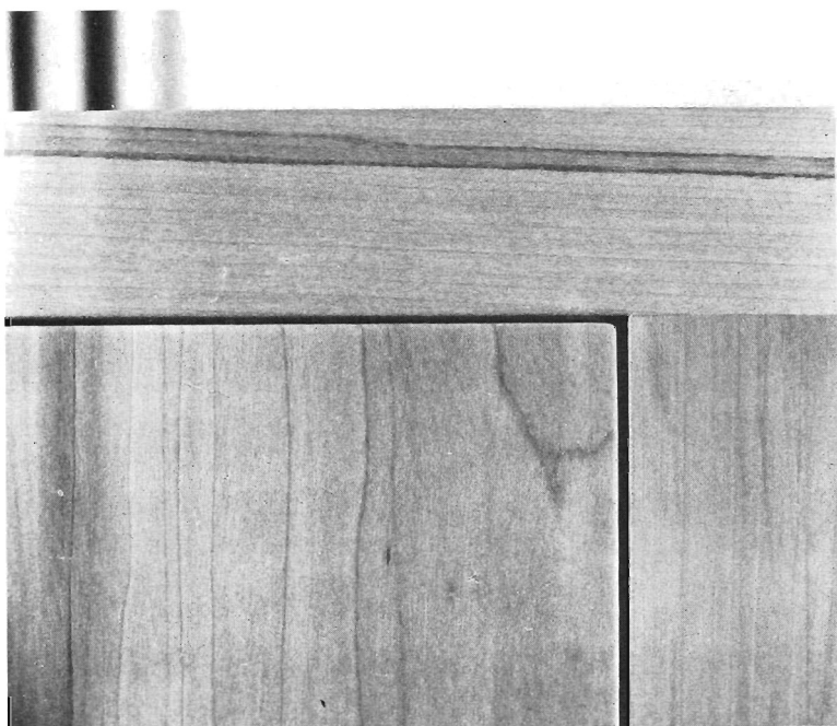
Detail of back glued and finished, before it is fitted to the cabinet.
