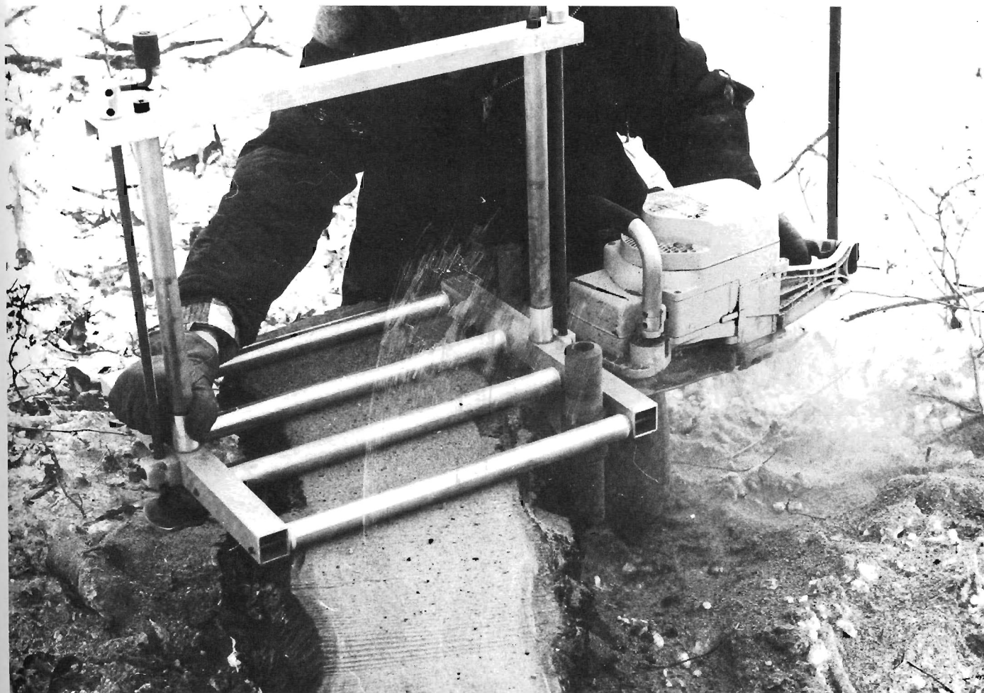
Portable mill with single motor is easily handled by one man. The saws shown here can be obtained from Robert Sperber, North Caldwell, New Jersey.
