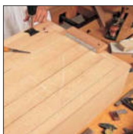
Installing Basic Hinges
