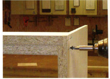
11 Install the sub rail. Secure it with staples or 1 1/4"-long No.8 drywall screws.
