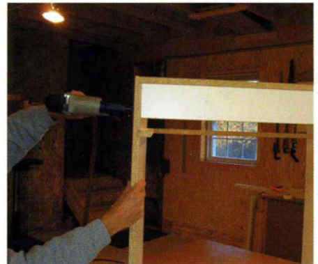
12 Install the nailer at the back of the cabinet.
