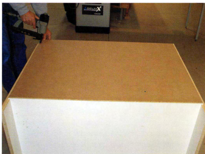
16 Attach the back with screws or staples.
