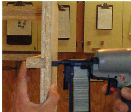
11 Install the drawer glide supports.
