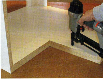
22 Turn the cabinet on its top and install the subrails.
