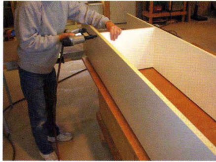
11 Continue up the cabinet and attach the divider to the side.
