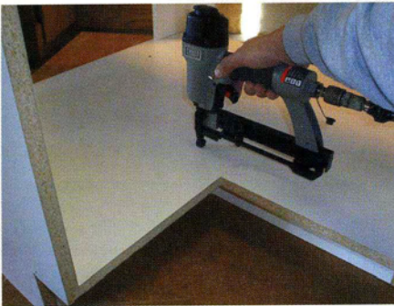
21 Install a couple of nails to secure the toe kicks to the base.
