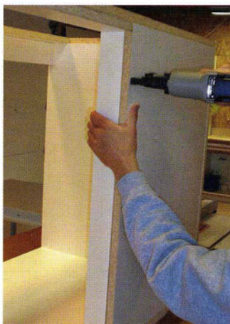
13 Attach the door support to the filler.
