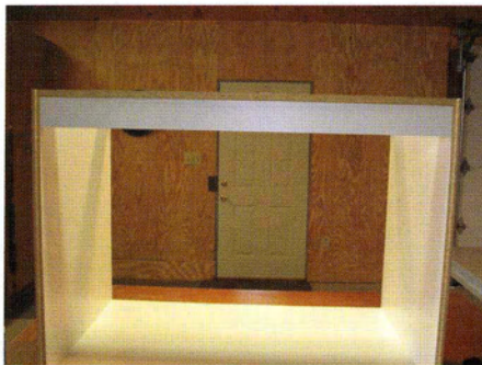
10 Install the nailer at the back of the cabinet.
