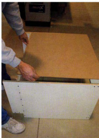
11 Lay the cabinet face down. The back should fit snugly into the rabbets. The back will help square the cabinet, so a good fit is important. You can use a framing square or measure diagonally from top to bottom. Repeat with the opposite corners. If the cabinet is square, both measurements will be the same. If the measurements are not the same, adjust the longest dimension by pulling the corners diagonally together until the cabinet is square.
