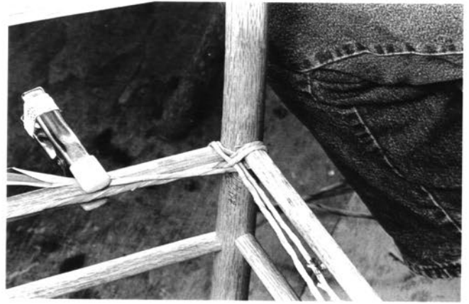
The wrap pattern after two rounds
