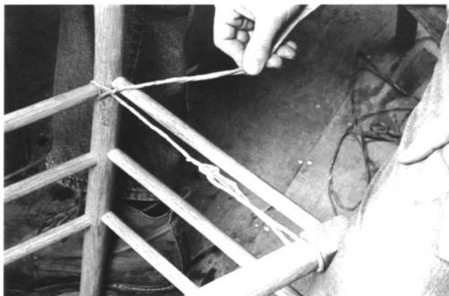
Observing the path of a single strand makes the rush pattern simple to understand.
