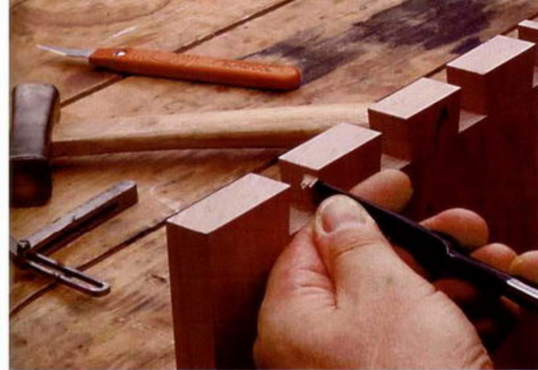
Photo A: Saw, then pare the tails with a chisel until you're satisfied they're right on. You'll use them to mark out the exact locations of the pins on the sides.
