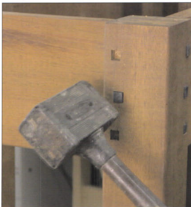
Making the plugs a consistent length, and pillowing the ends before inserting, speeds what can be a tedious process. Chamfer the back edges of the plugs and spread glue around the hole before tapping them in with a dead-blow hammer.
