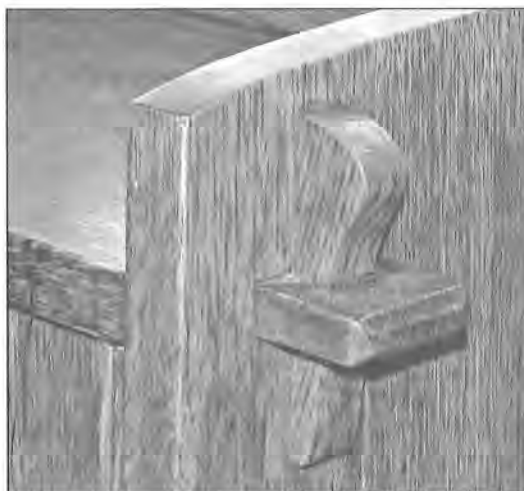
In some pieces, the through tenon extends and is held together with a wedge.
