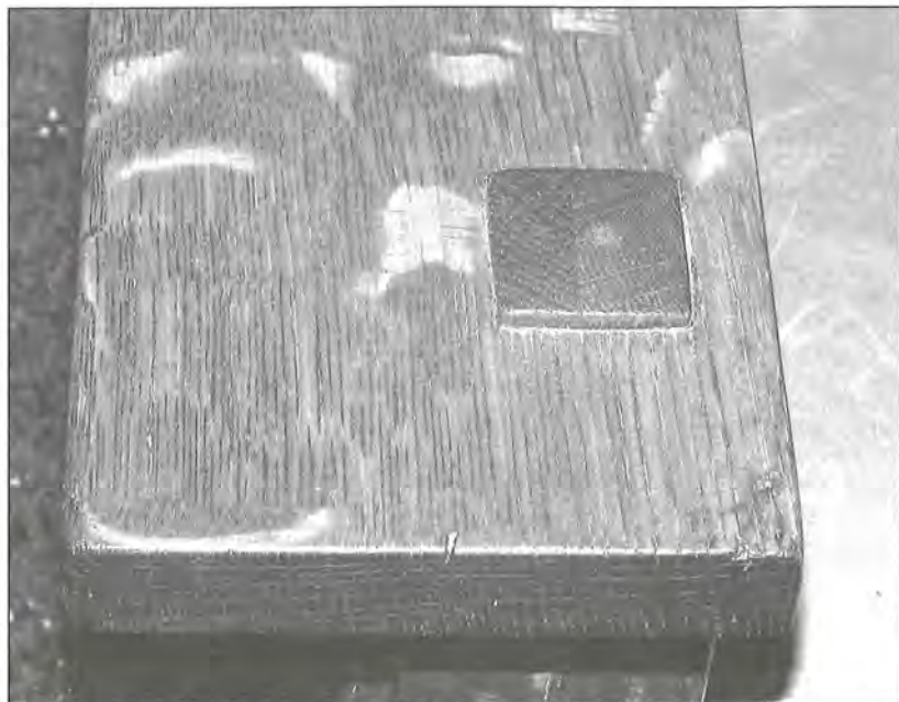
Edges are gently chamfered or rounded in original pieces. Variations in individual pieces indicate that this work was done by hand.
