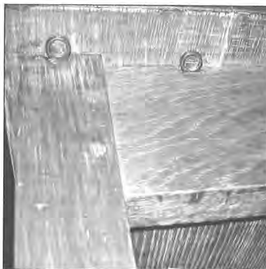
Tops were typically fastened with "table irons", figure 8 shapes held with screws.
