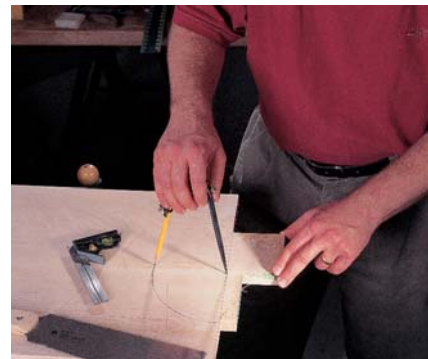
After cutting the bottom, lay out the radius (below).
