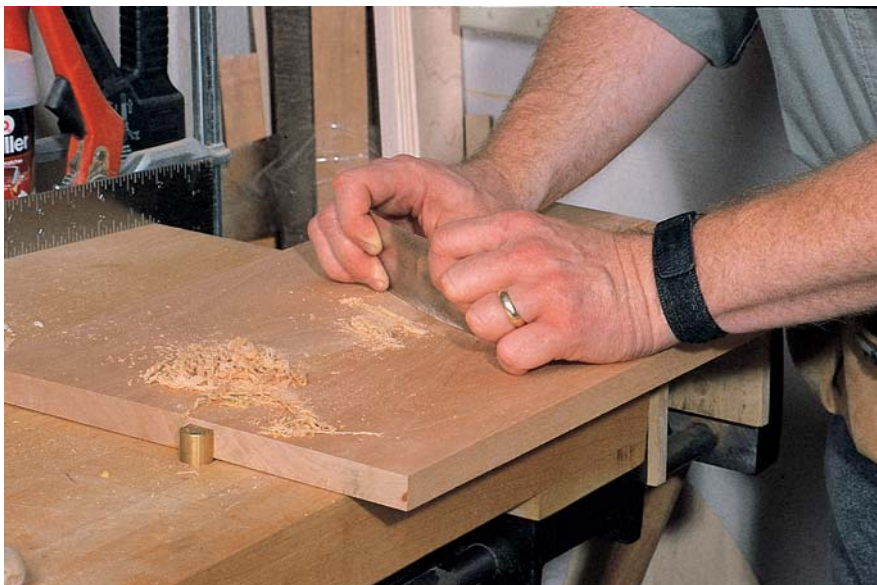
Glue up Your Panels. Taking some lumber from a friend's cherry tree, cut down, milled and air dried. I glued up two boards to make the top and ends for this bench. Some scraping of the joint is required after gluing. Try to arrange your boards so the joint between them is invisible.
