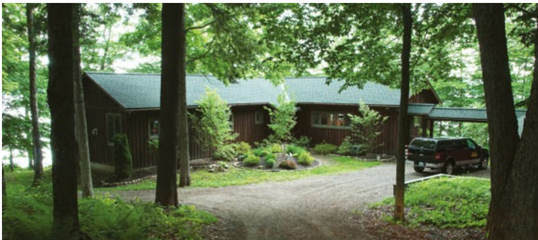
This 1980s ranch home gives little indication from the front of the extensive remodeling to the interior.
