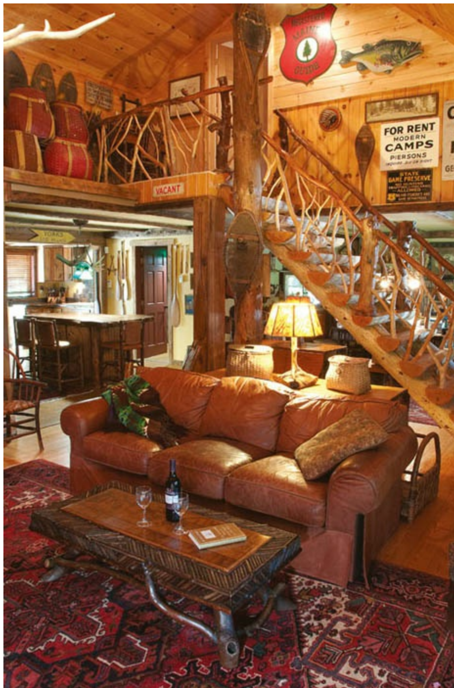
The wooden staircase leading to the upper floor was built using half logs from trees cut on the property, as well as newel posts made from apple trees.
