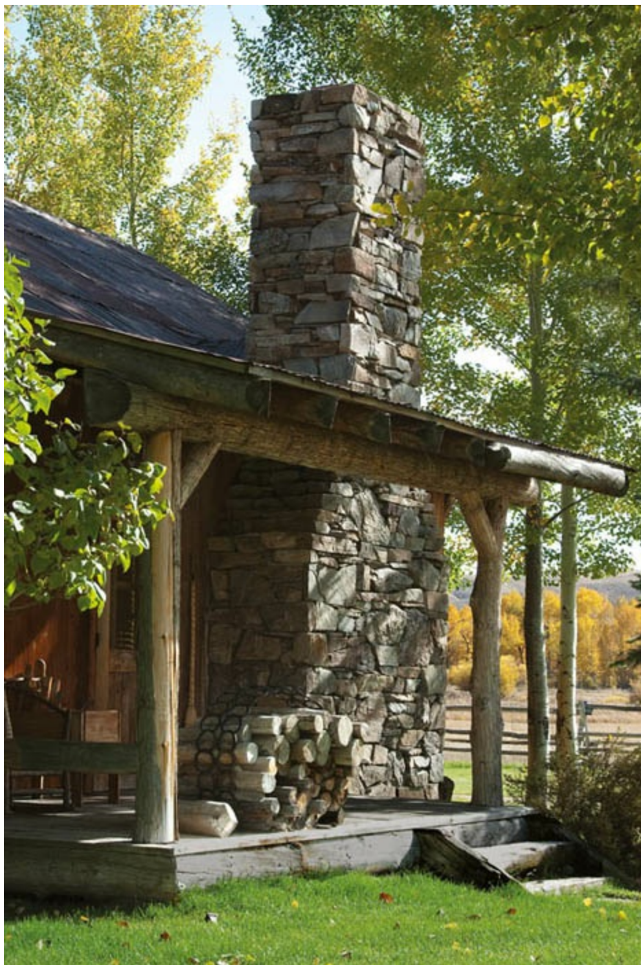
Many of the fireplaces were created by mason Phil Cox using locally quarried stones.
