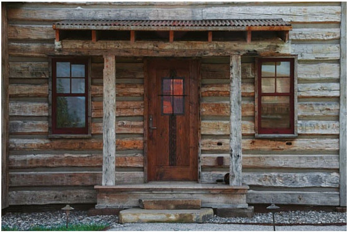
The cabin exterior includes hand-hewn slabs, recycled barn wood and cedar shingle roofing.
