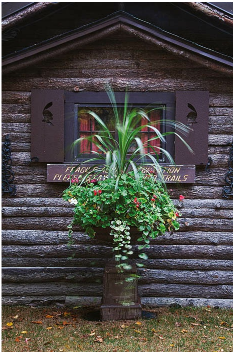
The cabin's exterior sports "pig siding," made from the leftover parts of trees after they're trimmed for lumber.
