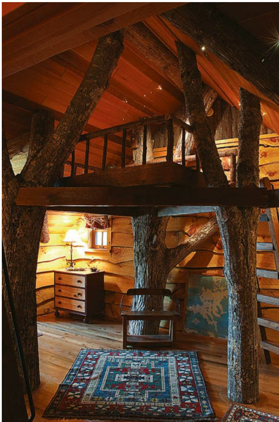
The tree fort bedroom's upper platform is supported by a forest of tree trunks.
