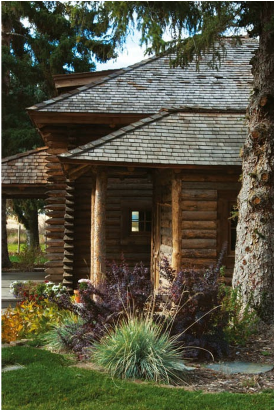
A view from the side of a smaller building, looking toward the main house, reveals different types of corner
