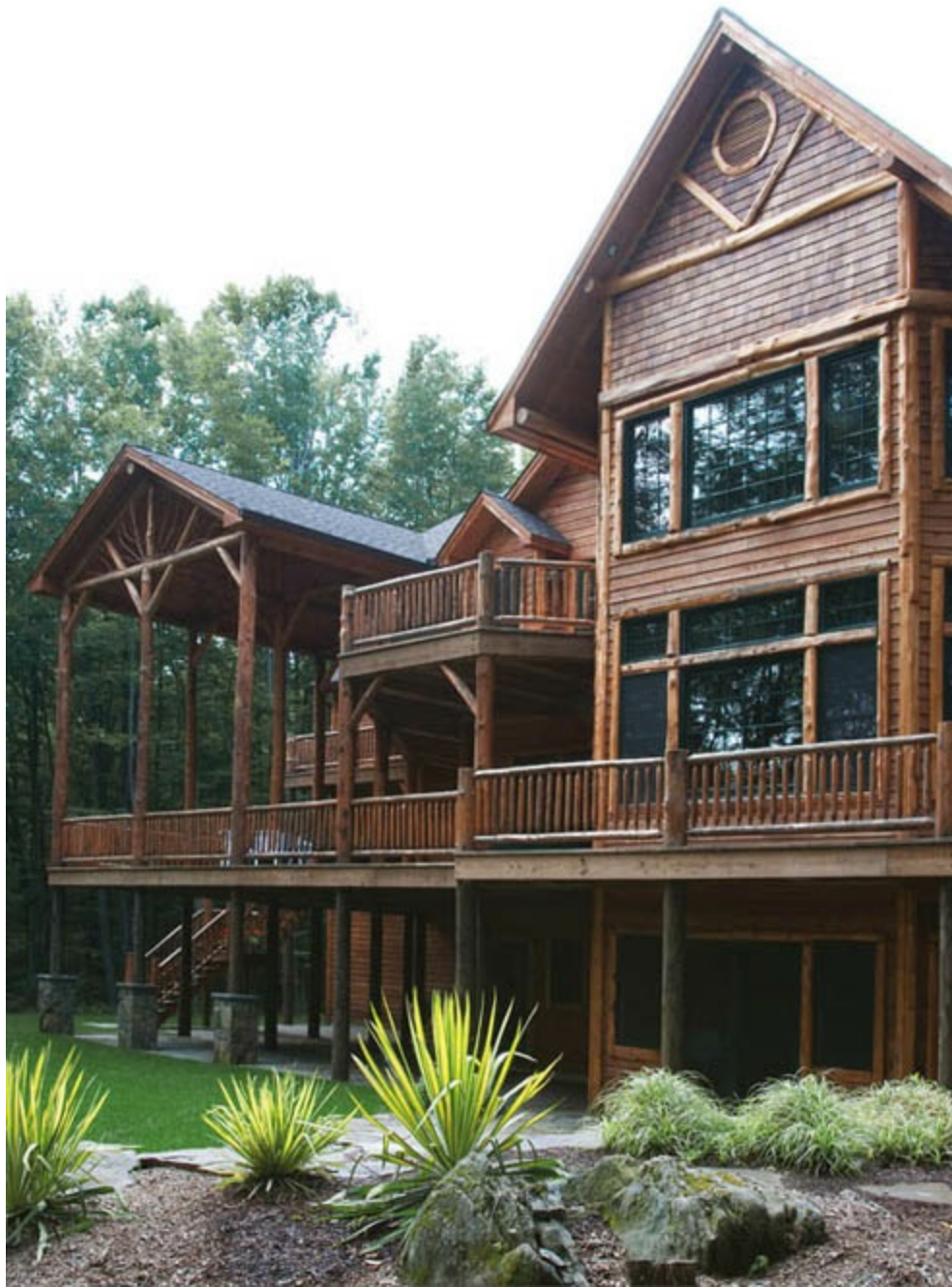
An interesting blend of horizontal boards, shake shingle siding and spit log details highlight the exterior face of the lodge.
