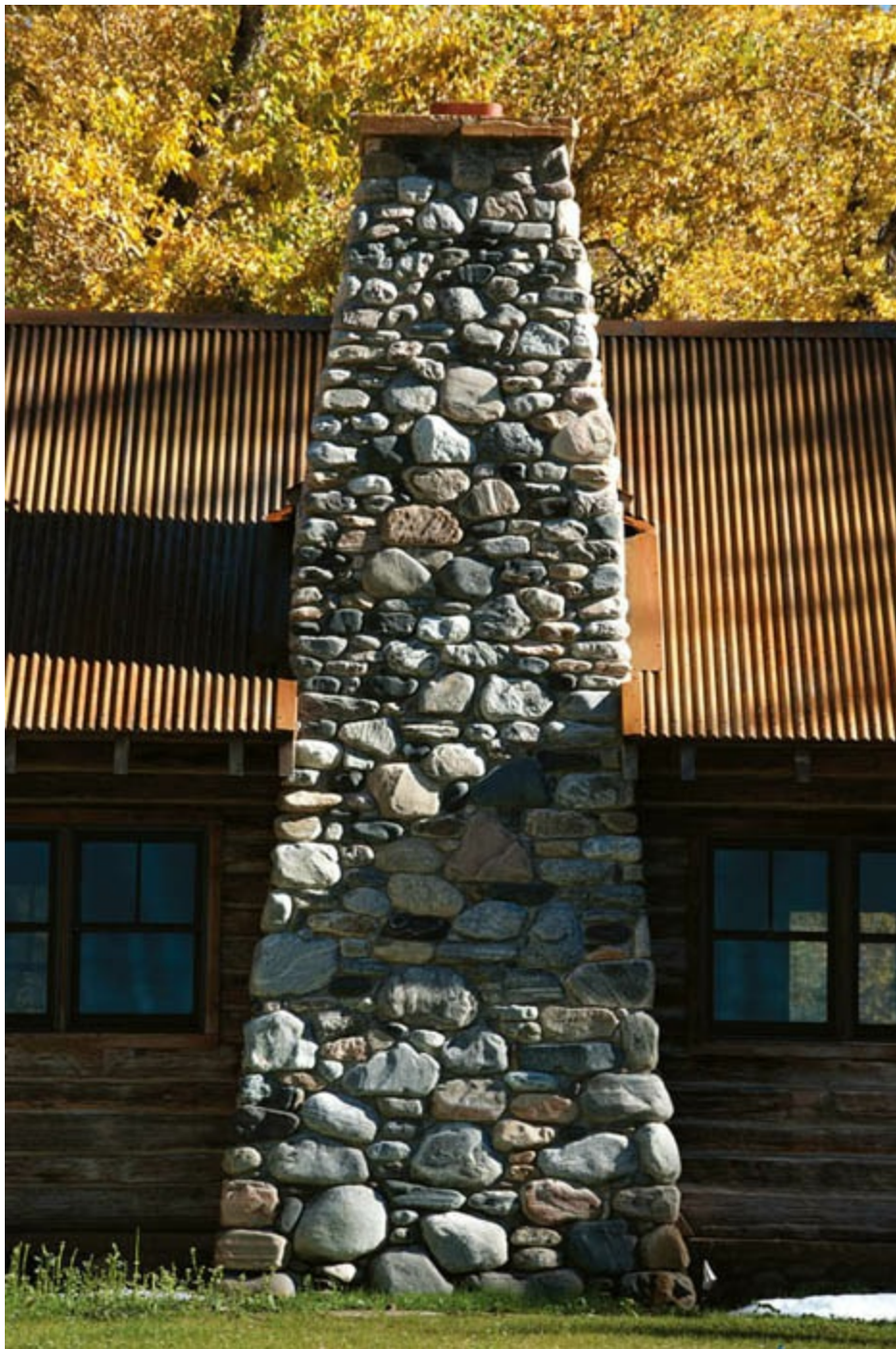
A tapered stone fireplace, built by Ron Davidson, dominates the exterior view of this side of the cabin.
