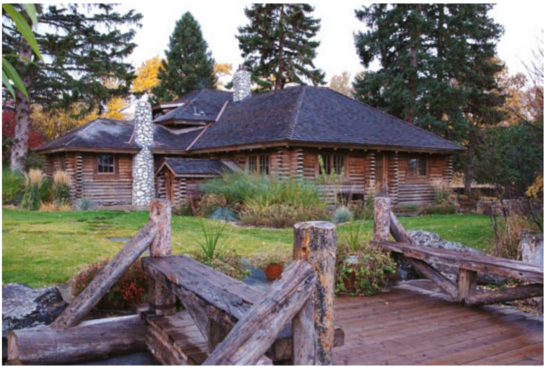
The original 1904 cabin is spectacular for its multiline roofing system and distinguished corner configurations.
