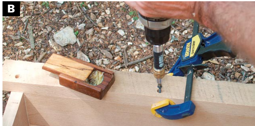
ADD THE HINGE-MOUNTING STRIP at the back of the chest, using glue and countersunk wood screws to hold it in place. A bit of wax on the screws will ease their passage into the wood.
