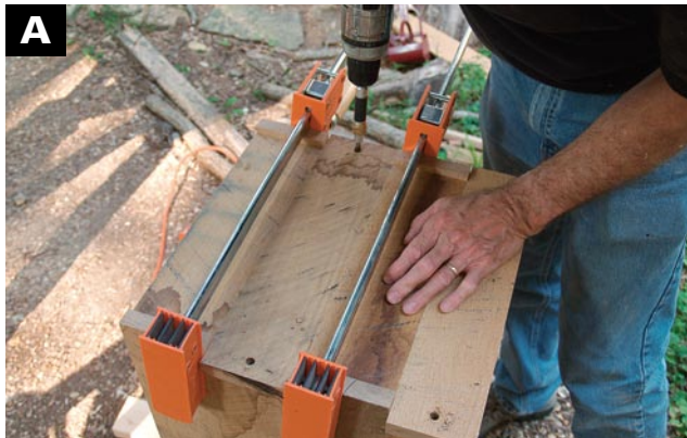
USE CLAMPS TO HOLD THE FRONT and back tight to the ends as you drive screws in place. I countersink the screws deep enough that I can use walnut dowels to fill the holes and hide the screws.
