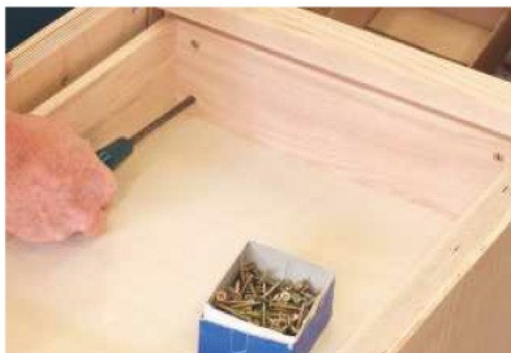
34 With the drawer fitted, locate the drawer front in its aperture and drive screws into it from inside
