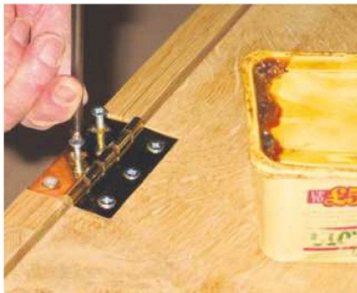
23 Applying a little grease to each screw thread will help them to drive in easily.
