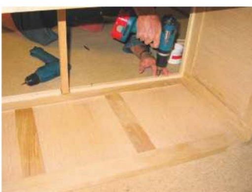
15 Screw and glue softwood battens to the lower rails to support the base panel
