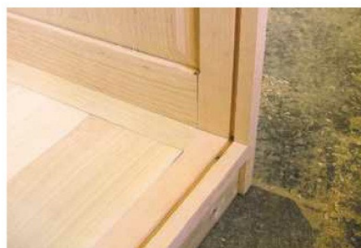
20 Form a groove in the end frames and the base panel to take the plywood back
