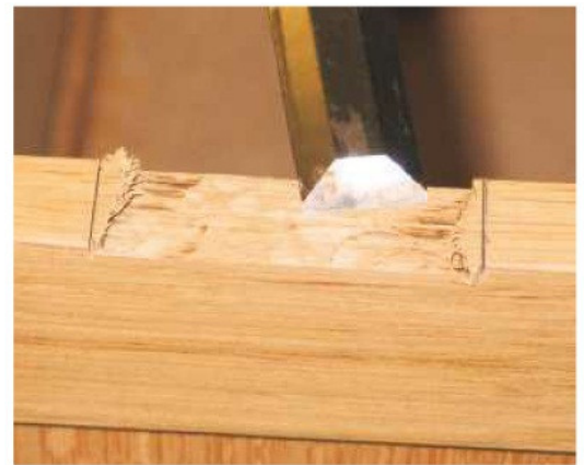
22 Chop out the waste from each hinge recess to the required depth using a sharp chisel.
