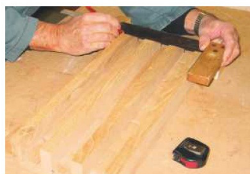
8 Mark out the mortise hole positions on the four legs in one operation
