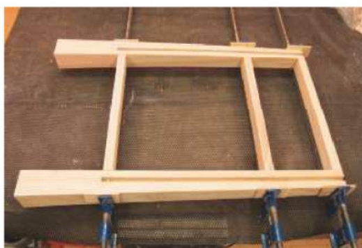
15 Glue and cramp up each pedestal front by assembling two legs and three rails
