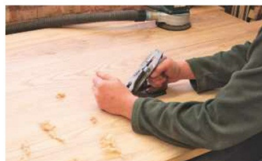
40 When the glue has dried, flatten all the joints with a sharp plane
