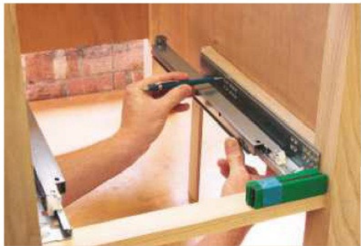
19 Position the drawer runners accurately and mark their fixing holes
