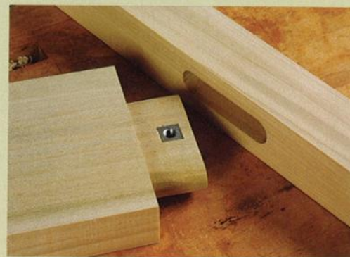
HIDDEN NUT. The nut is inset into the tenon on the head or foot rail and faces away from the side rails.
