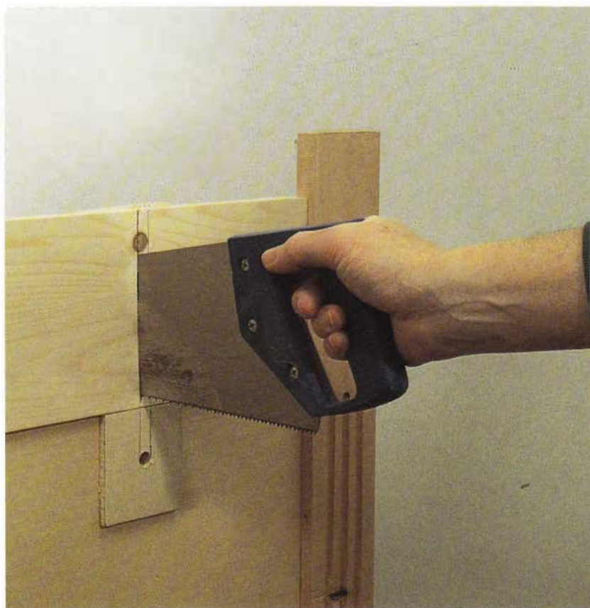
FIG 10.9 Cutting the slots with a panel saw.
