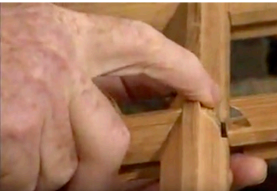
The Woodwright’s Shop, Roy Underhill, points out the sash bars (muntins)—moldings which have a mitered and overlapping joint.
