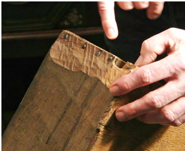
Axe marks and crude thinning to support nailing of drawer back to sides on 17th century chest drawer. Photo courtesy of Dale Ausherman, with permission of Adam Bowett.
