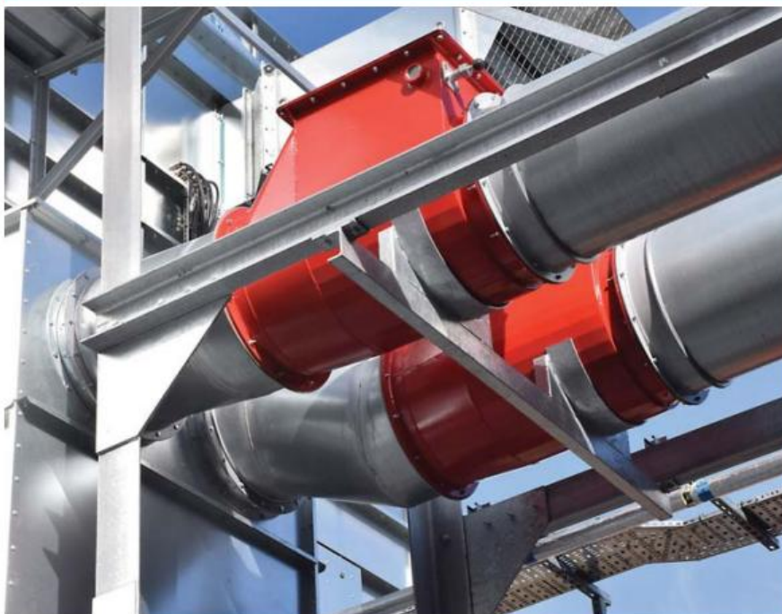
In the event of an explosion, back pressure explosion isolation valves are designed to prevent the effects of a pressure wave and flames travelling back along ductwork and into the factory.
