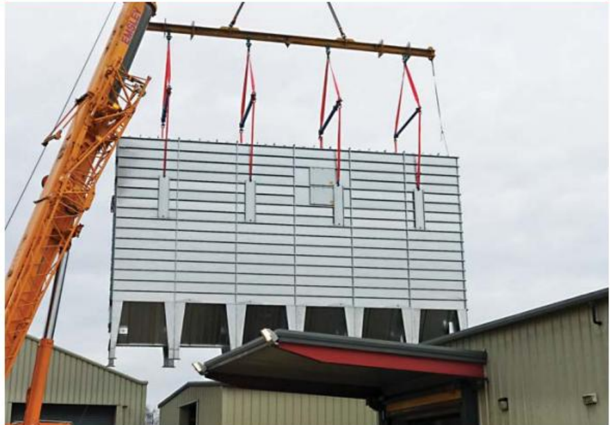
One of the ECOVAR VALIDUS filter units being craned in between buildings at JJO.
