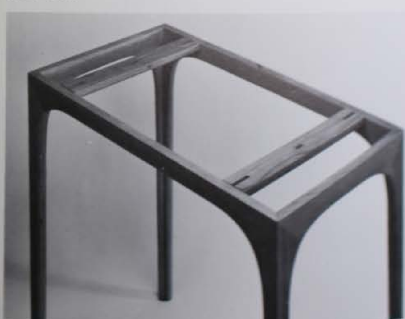
D. Tabletop support stringers are slotted for screws and mortised into the ends of the long aprons. Screw slots allow the top to expand and contract without bowing or cupping. Mortises are routed before tabletop frame is completely assembled.
