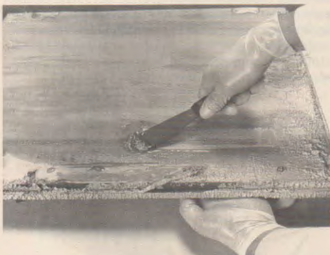
Fig. 48-28. After washing the surfaces, rub with steel wool. (Benjamin Moore)
