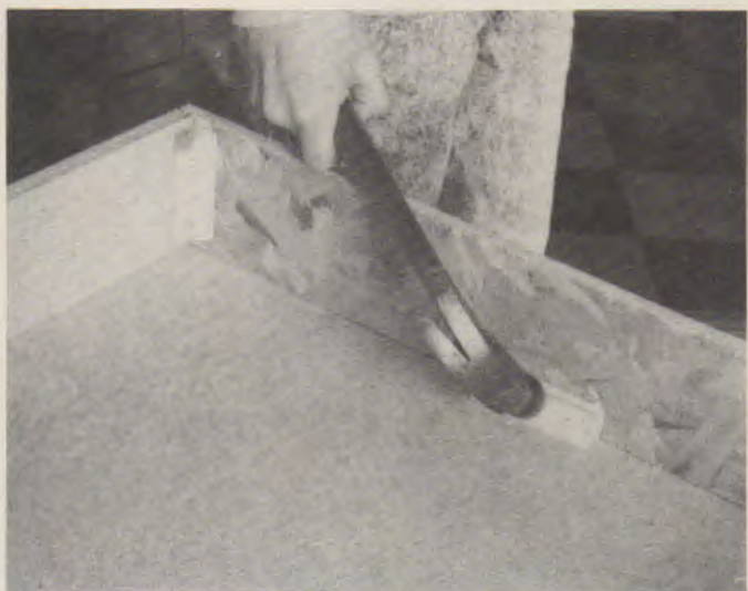
Fig. 49-46. Toe board glued with blocks and fastened with brads.
