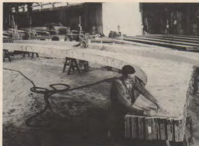
Fig. 34-11. This lamination will be an arch for a cathedral ceiling. (Forest Products Laboratory)
