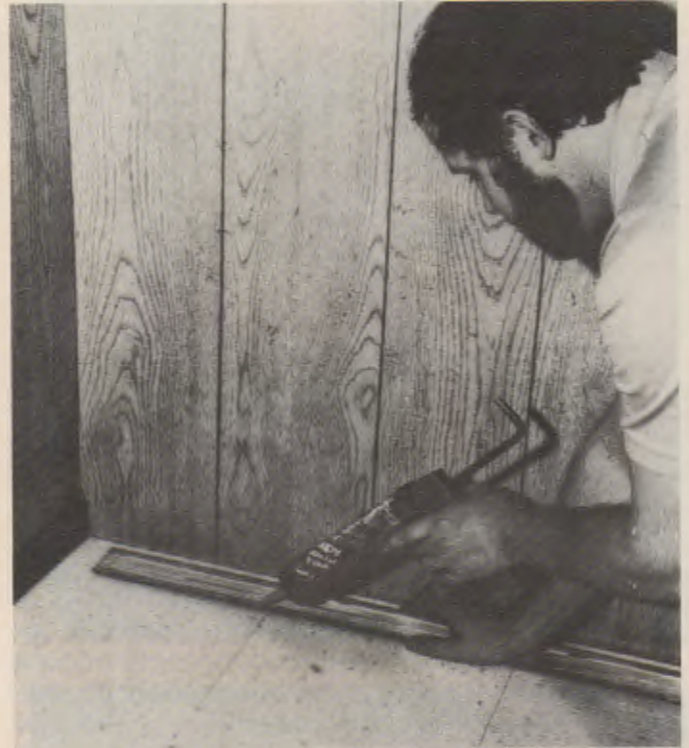
Fig. 32-13. Install vinyl trim, base, and mouldings with a vinyl adhesive. (Franklin International)
