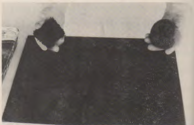
Fig. 47-21. Stippling gives a textured appearance. It can be done with a sponge or nylon scrubbing net.
