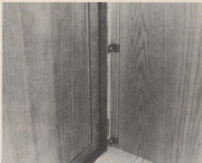
Fig. 49-45. The face frame may be attached to clips set in a groove in the cabinet side.
