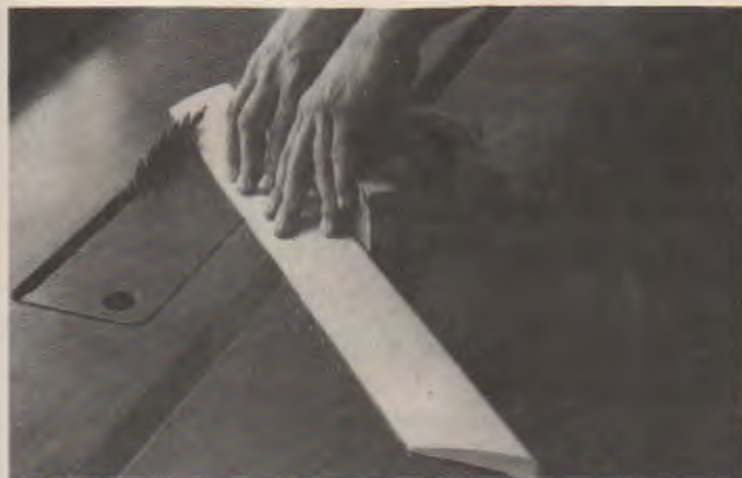
Fig. 21-19. Sawing a miter. The guard has been removed to show the operation.
