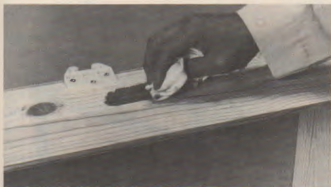
Fig. 47-5. Test stain on a hidden surface before applying it elsewhere.
