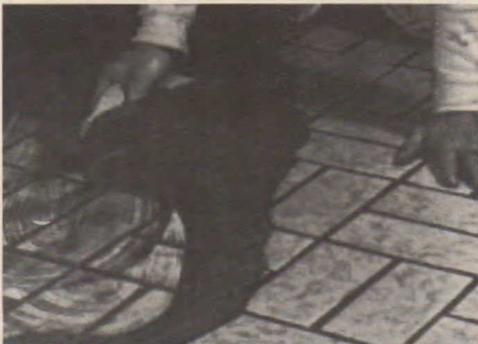
Fig. 32-15. Steps in applying grout. A—Spread grout into spaces between tiles with a grout float. B—Wiping off excess grout with a wet sponge. (Franklin International)
