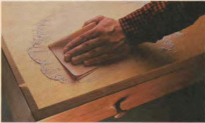
Fig. 48-1. Between-coat deglossing with 180 grit abrasive paper. (Carver-Tripp)
