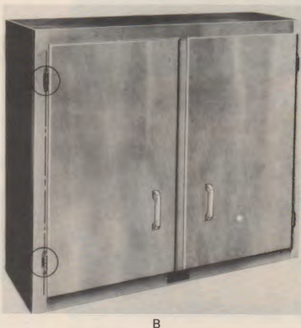
Fig. 41-9. A—Install lip-edge doors with nonmortised hinges. (Liberty Hardware) B—Make sure the barrels are aligned so that the door does not become hinge bound. (Brodhead-Garrett)
