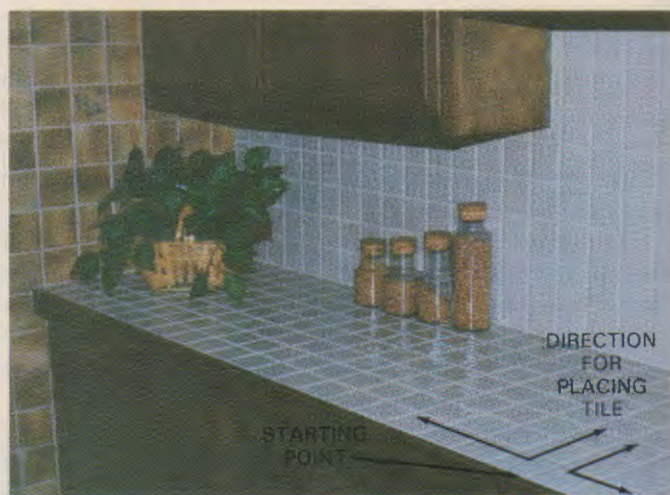
Fig. 15-36. A one edge tile layout begins at the front edge. This type of layout is common for countertops.
