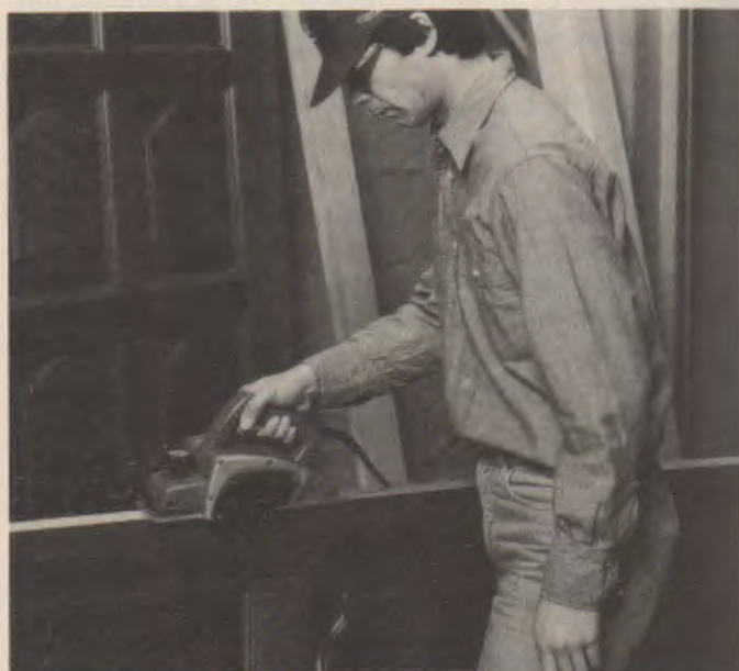
Fig. 24-19. Portable power plane are useful for on-site architectural woodwork. (Rockwell)
