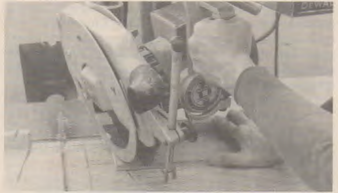
Fig. 21-29. Compound mitering with the radial arm saw.
