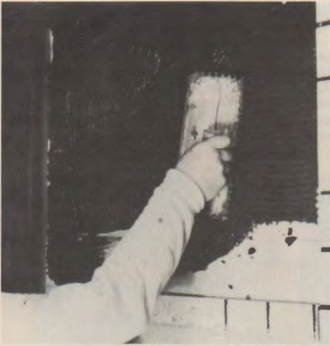
Fig. 32-14. Apply tile adhesives with a notched trowel. (Franklin International)
