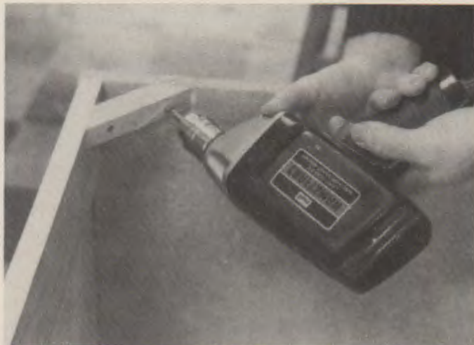
Fig. 49-47. Corner blocks position and secure the cabinet top.
