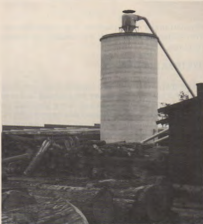
Fig. 11-3. Logs stored on land are stacked and kept moist to prevent premature drying. (Hoge Lumber Co.)
