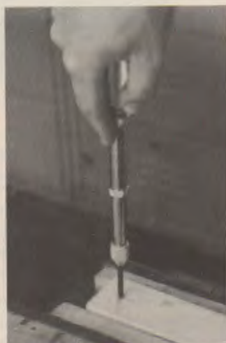
Fig. 25-12. Drill points fit in a push drill. They make holes for screws, brads, and other purposes. (Stanley)
