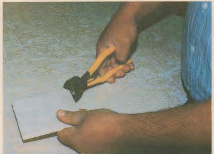
Fig. 15-39. Tile nippers chip off bits of tile for irregular shapes.
