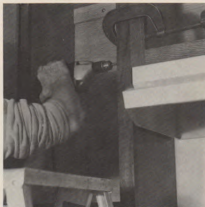
Fig. 49-32. Hang the cabinets, then fasten them to each other. (Jae Company).
