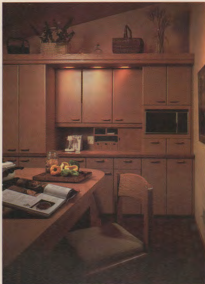
Fig. 14-13. The surfaces of the cabinets, countertops, and table are covered with plastic laminate. The laminate covers particleboard construction. (Sterling Engineered Products, Inc.)
