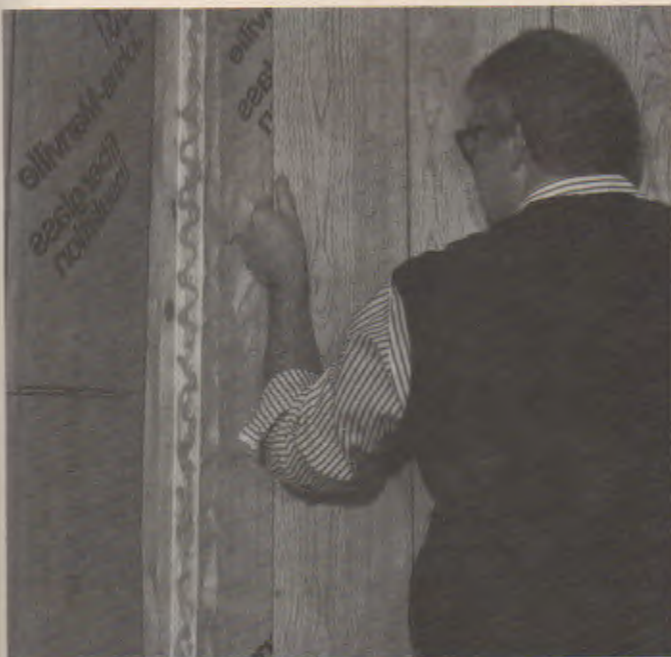
Fig. 32-12. Prefinished plywood panels are attached with panel adhesive which has been applied to wall studs. (Franklin International)
