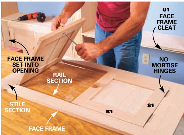
**14 INSTALL** no-mortise hinges (see Buyer's Guide) on the stiles and the door edges before installing the face frames in the bookcase. Make sure to leave 1/16-in. clearance between the doors and the face frame. If necessary, use a belt sander to fit the doors precisely in the face frame openings. Attach the knobs to the doors, hang them on the hinges and nail the assembly to 3/4-in. x 3/4-in. pine strips set back and glued into the cabinets.
