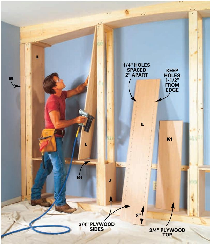
**7 RIP** 3/4-in. oak plywood to 11-7/8 in. and then drill 1/4-in. holes for standard shelf clips. Use a strip of 1/4-in. Peg-Board as a template for the shelf clip holes. Drill the holes, positioning the template to the bottom of each piece to ensure the shelves will be level when installed.
