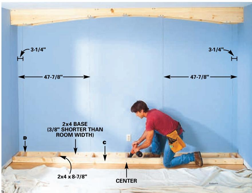
**4** **BUILD** the 2x4 base as shown in Detail 2, p. 39, and screw it to the floor with 1-1/2 in. x 1-1/2 in. steel angles. Space the 2x4 blocks so the vertical uprights marked on the walls will stand directly over them later.
