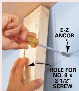
**6** FASTEN the 2x4s to the wall as shown. Use E-Z Anchors (photo at left) if wall framing isn't available behind the 2x4s. Scribe the 2x4 supports to fit under the curve. Note that the 2x4 supports on each side wall are set back 3/4 in. behind the 11-7/8 in. mark.
