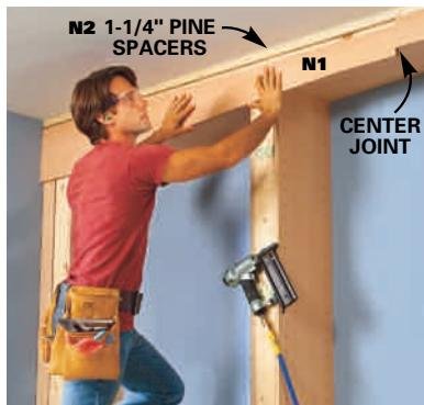
**8 NAIL** a 3/4-in. x 1-1/4 in. filler to the top of the apron assembly, then nail the arched 1x10 oak pieces (cut in half to fit) to the apron assembly. Scribe the pieces to the side walls if necessary. The center joint will be covered by the keystone trim later.
