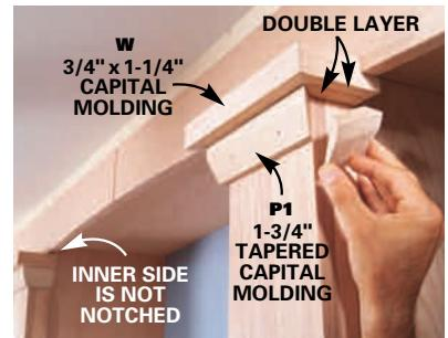
**19** FIT the capital moldings around the tops of the columns. Use a double layer at the top to build out the surface and notch these layers around the lower edge of the curve. Place the 3/4-in. x 1-3/4 in. tapered molding directly below and nail it in place with the brad nailer.
