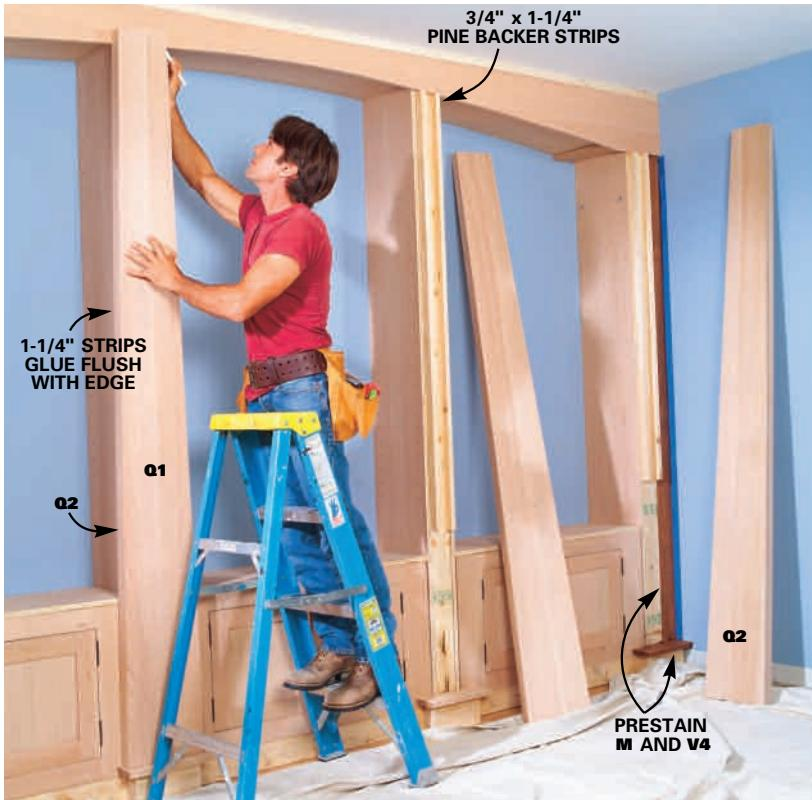
**18** SET the columns onto the base caps and mark each side of the column where it meets the upper arch. Be sure the column is centered on the 2x4 support behind. Build up the upper face of the 2x4 supports with 1-1/4 in. deep strips to ensure the column lies 1-1/4 in. in front of the oak arch. Nail the columns to these strips and to the face of the 2x4 and face frame below with 10d finish nails.
