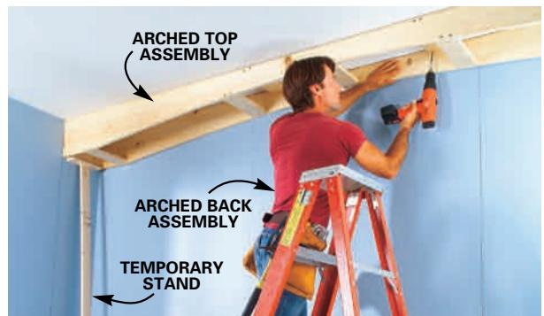
**3** **LIFT** the apron assembly to the ceiling and build a temporary stand for each end to keep it tight to the ceiling as you screw it to the framing. If framing is difficult to find in key areas, use wall anchors (bottom photo, p. 39) to fasten it to the ceiling and side walls.
