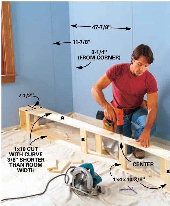
**2** **CARRY** the two arched aprons into your room and screw 1x4s between them as shown with 1-5/8 in. wood screws. Drill pilot and countersink holes to avoid splitting the wood. Be sure to complete the layout lines on the wall (Photo 4 and Detail 2, p. 39).
