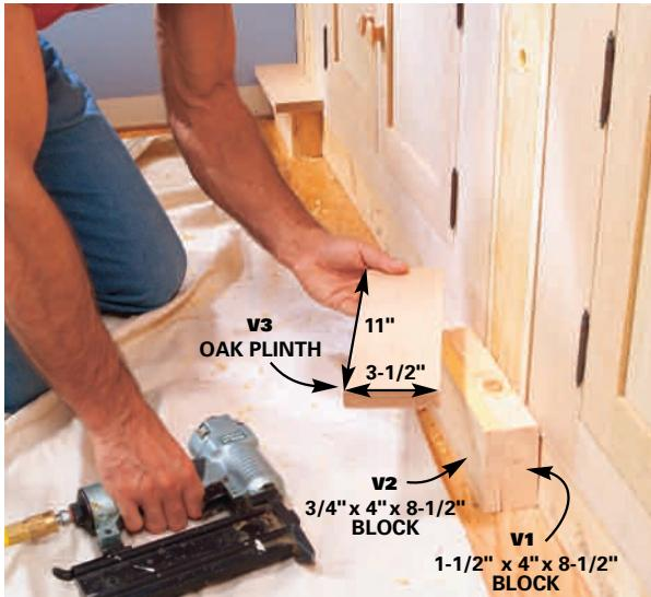
**17** RIP 2x6 and 1x6 pine to 4-in. widths and nail them to the base assembly at the center of each 2x4 vertical support. These pieces will support the base cap. Next, wrap these supports with 3/4-in. x 4-in. oak base pieces and continue installing these base pieces between the column bases.
