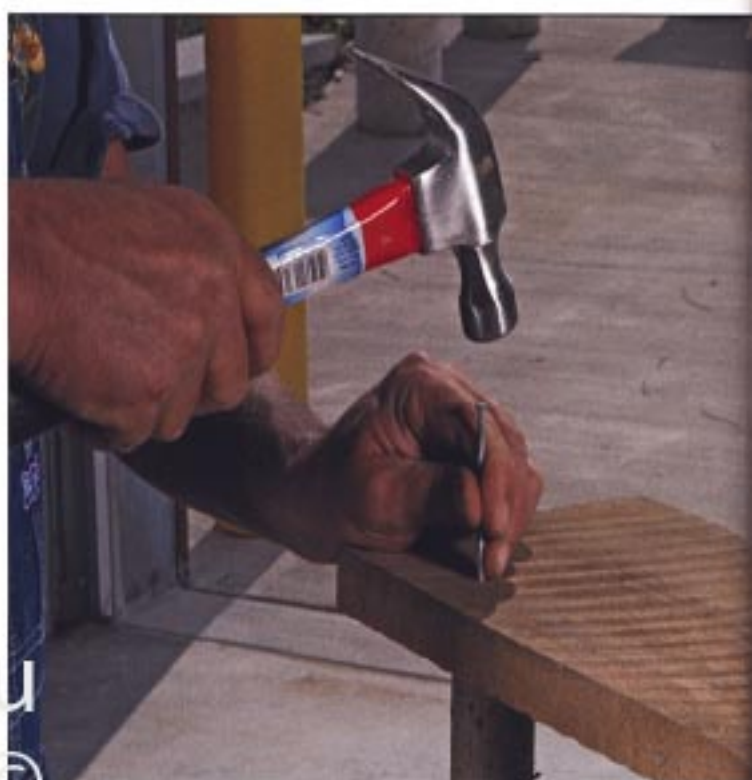
Using 10p nails, nail one side through the top into the leg.
