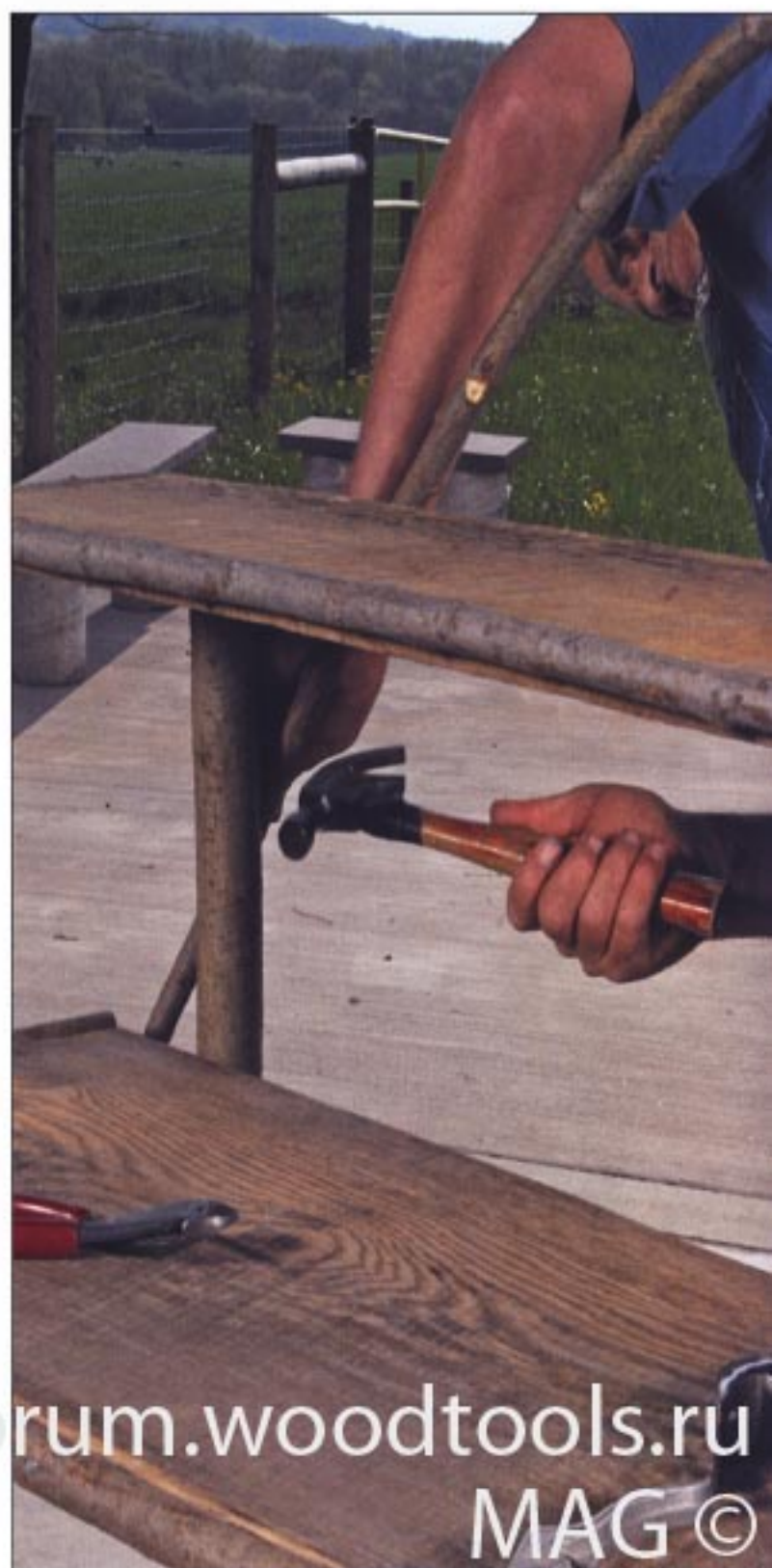
Secure it with a 6p nail.
