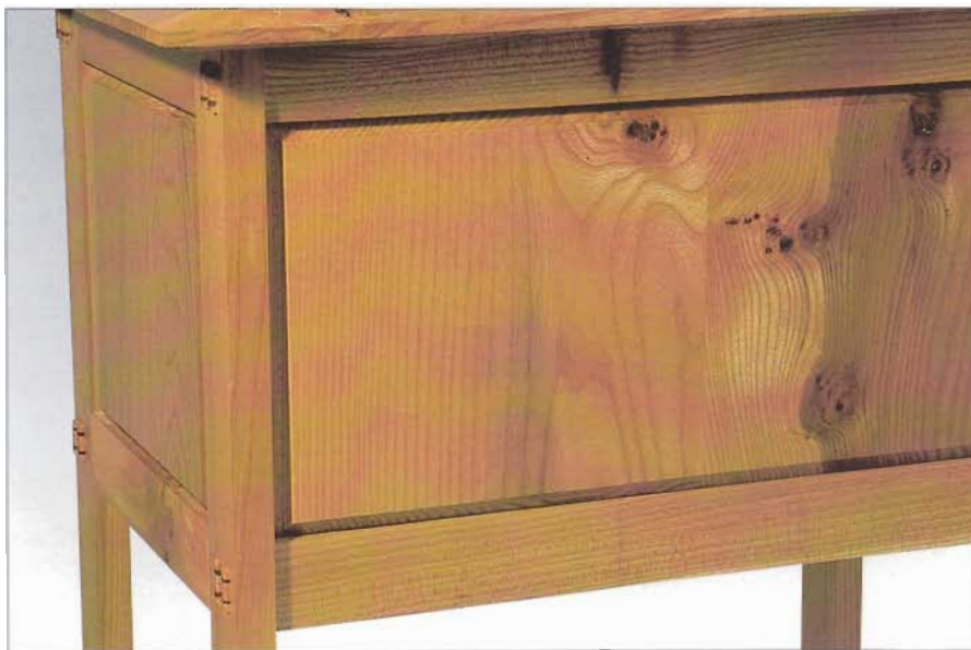
The back panel is solid and grooved into the rails
