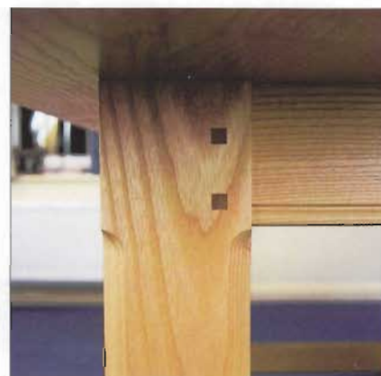
Decorative detail: plugs, chamfers and beading
