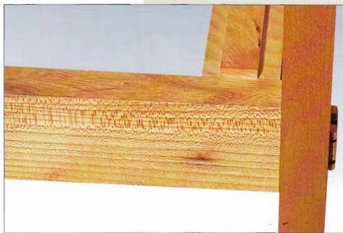
Drawer runner detail showing strip glued to give extra smooth operation
