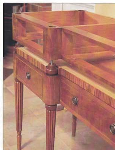
Top carcass in position on rods
