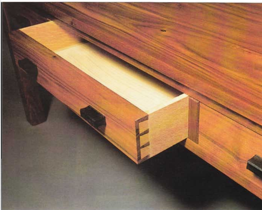
Drawer construction is traditional, complete with slips and quarter-sawn oak sides
