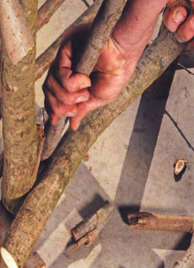
Using a 4p nail, secure the thick end of the willow to the back of the front leg.
