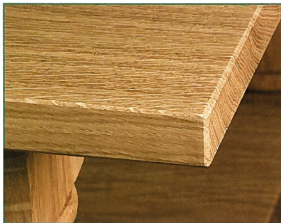
• Hand-planed chamfer on table top
