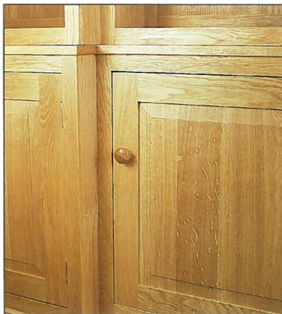
• Traditional fielded panels on the doors
