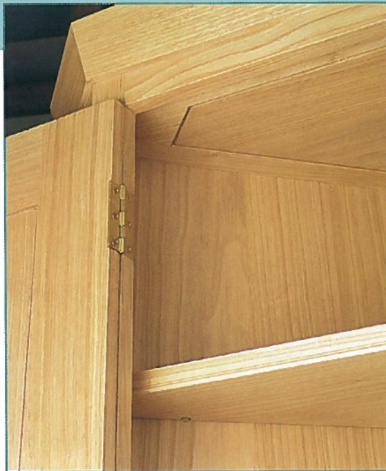
• Interior of door panel and bead moulding on the shelf add interest
