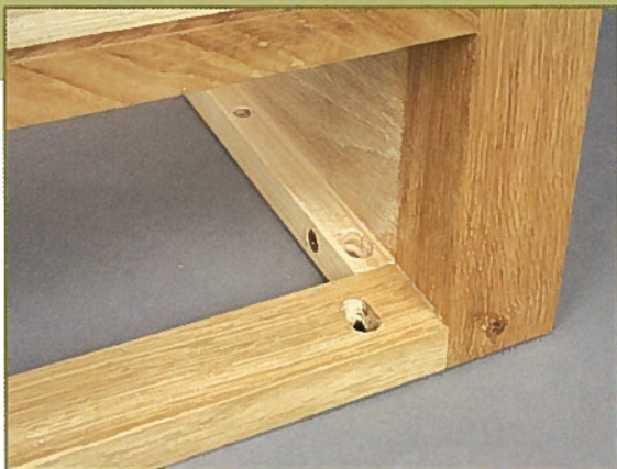
• The slots for fixing at the leg end
