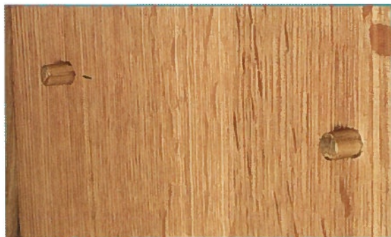
• Wooden pegs are used to support the adjustable shelves
