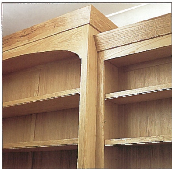
• View from the ground, showing cornices and curved arch on main carcass
