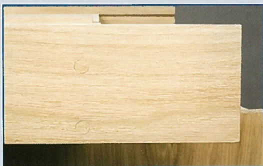
• The backs are screwed and plugged
