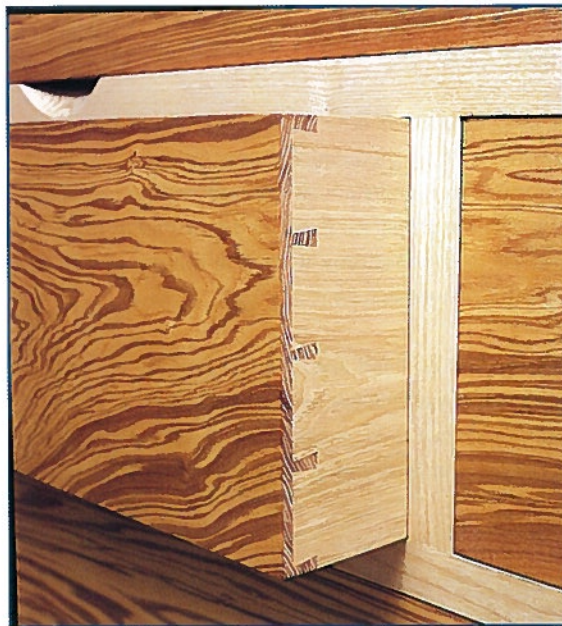
• Traditionally lapped dovetails on fronts
