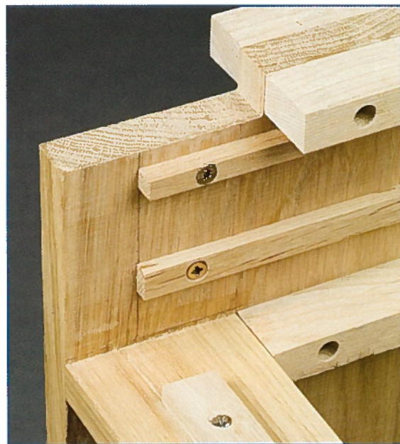
• Runners for the extension and the drawer that supports it
