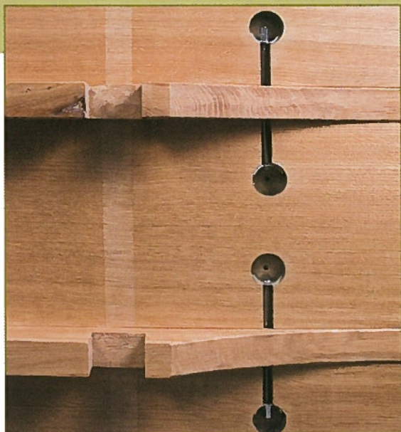
• The worktop bolts that lock the top together
