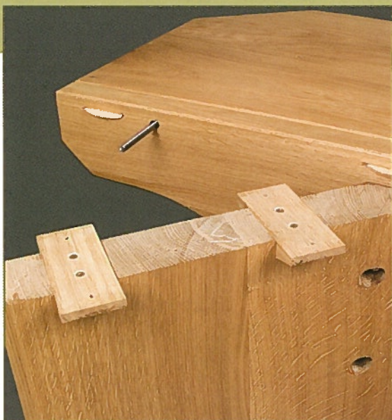
• Biscuits help align the top while bolts hold it all together
