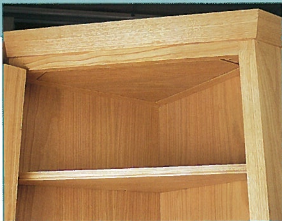
• Interior detail is important – there is a neat shadow line around the top panel
