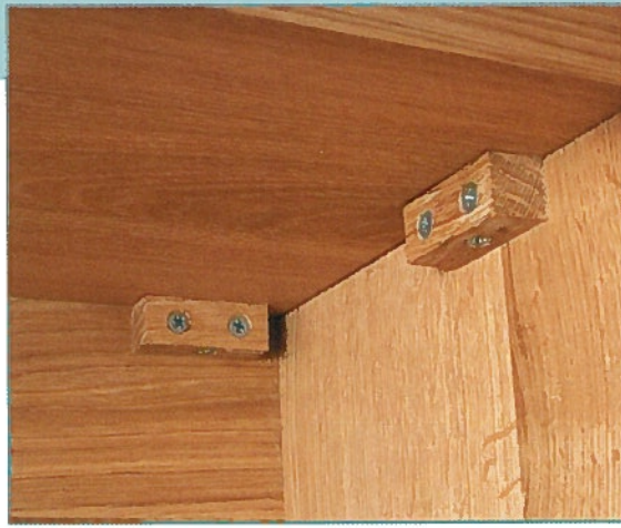
• Fixing blocks on the top
