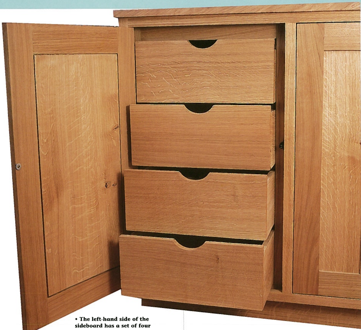
• Runners allow deeper drawer fronts and give clean visual lines, as there are no dividers
