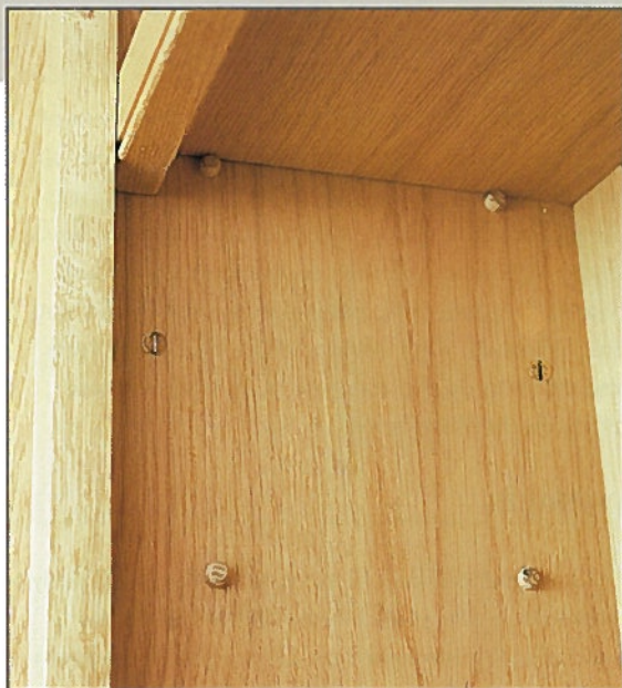
• Cabinets are screwed together – note the wooden dowels to support the shelves
