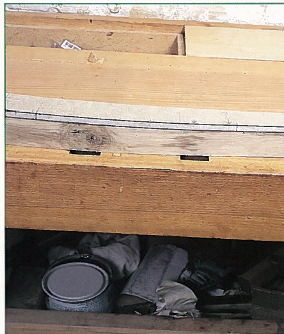
• Positions of joints are marked from these onto the legs
