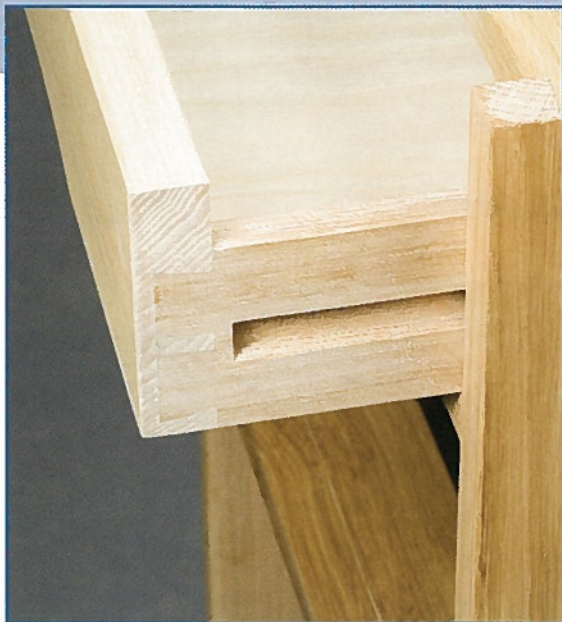
• The left-hand drawer acts as a support for the extension
