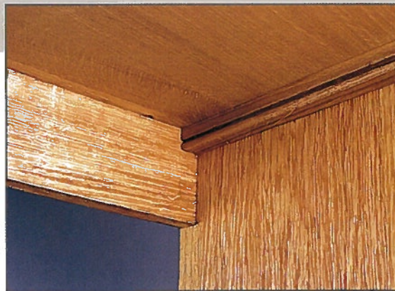
• Batten supporting back of the top carcass
