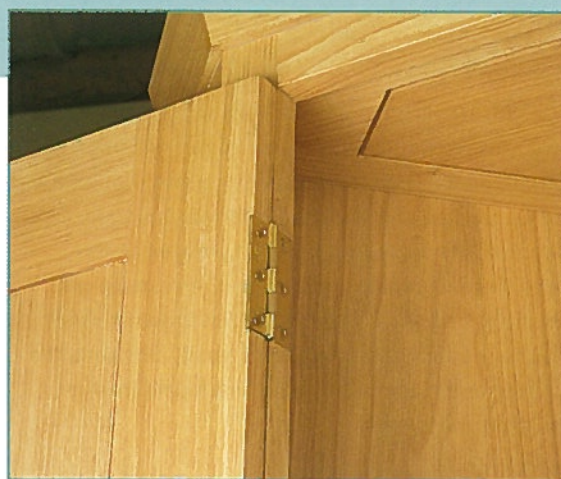
• The hinges are recessed into door style and cabinet frame
