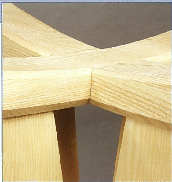
• Close-up of the cross-halving joint on the foot
