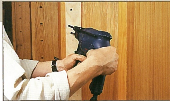
• Drilling the holes for the adjustable shelving
