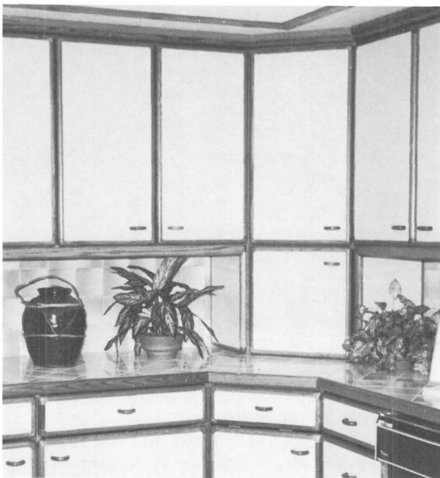
Illus. 239. This corner appliance garage hides small kitchen appliances and yet keeps them at counter level for easy use.
