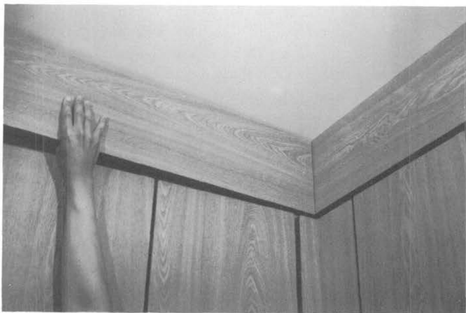
Illus. 237. You need to use a trim strip with style-one modules to hide the space between the cabinets and the ceiling. A trim strip is made from the same material as the doors. Use plastic T moulding along its lower edge. Scribe the top edge to fit the irregularities of the ceiling. To attach the trim strip, drive 1¼" dry-wall screws through the front filler inside the cabinet into the back of the trim strip.
