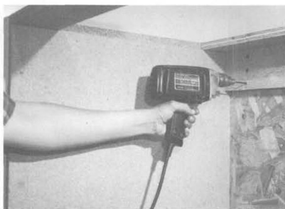
Illus. 232 (left). Use cedar shingles or tapered wedges to shim the bottom of the modules so that they are all even at the top and level. After shimming, tighten the C-clamp to hold the modules together while installing screws in the sides to attach them to each other. Illus. 233 (right). Attach the module to the wall with 3"-long dry-wall screws, which are driven through the nailing strip into wall studs.
