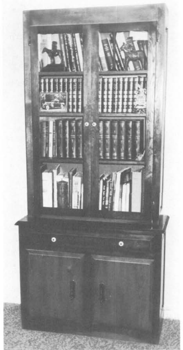
Illus. 167 (left). These raised panel doors give a traditional look to built-in cabinets. Illus. 168 (right). The glazed doors on this bookcase protect the contents while also allowing them to be seen.
