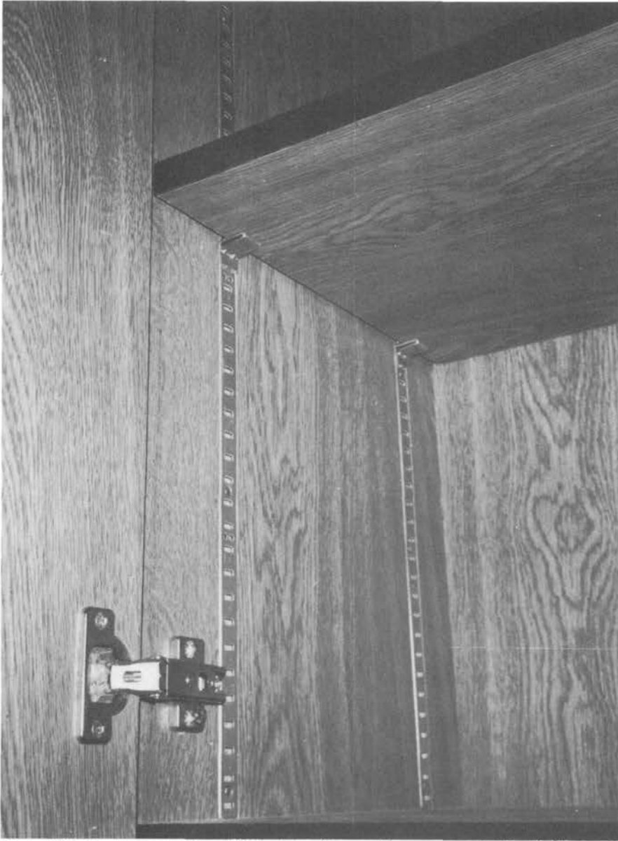
Illus. 157. Metal standards and brackets offer a wide range of shelf positions.
