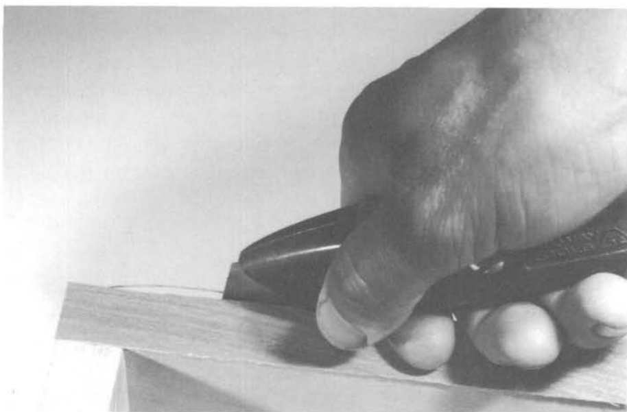
Illus. 17. Use a razor knife to trim the edges of the tape flush with the sides of the board.
