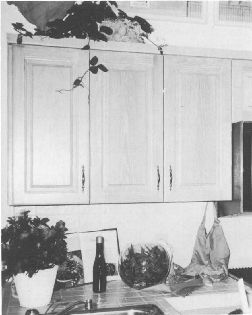
Illus. 206. Style three: Panel doors give this style a traditional look. The doors in the photo were made using a matched set of router bits to raise the panel and cut the sticking and coped stub-tenon joints. A matching piece of moulding acts as a cornice across the top. The cabinets do not extend to the ceiling; the area in between can be used for display, as shown here.
