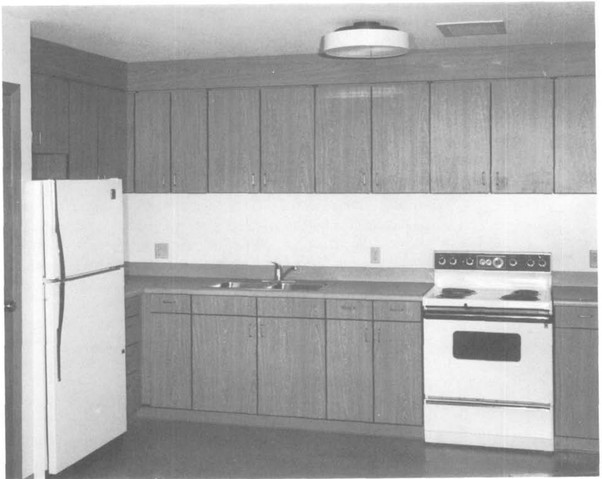
Illus. 198. These cabinets are too long to be moved in a single piece. Instead, they are built in standard-size modules and assembled in place.
