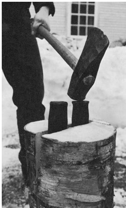
HALVE THE BILLETS. SET ONE or two wedges in the center, and drive them to open the billet. Sometimes, a solid blow will spilt a billet cleanly.
