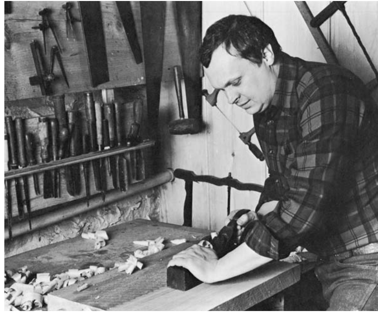
CLEAN UP THE ROUGH FACES of the seat blank so you can decide which is the best face for the top surface.
