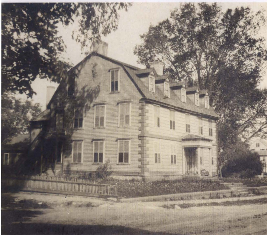
FIGURE 1.8. Bowers House, Somerset, 1760–65. Partially destroyed by fire, the house was demolished in 1957. Photo, ca. 1900, courtesy of Winterthur Archives.
