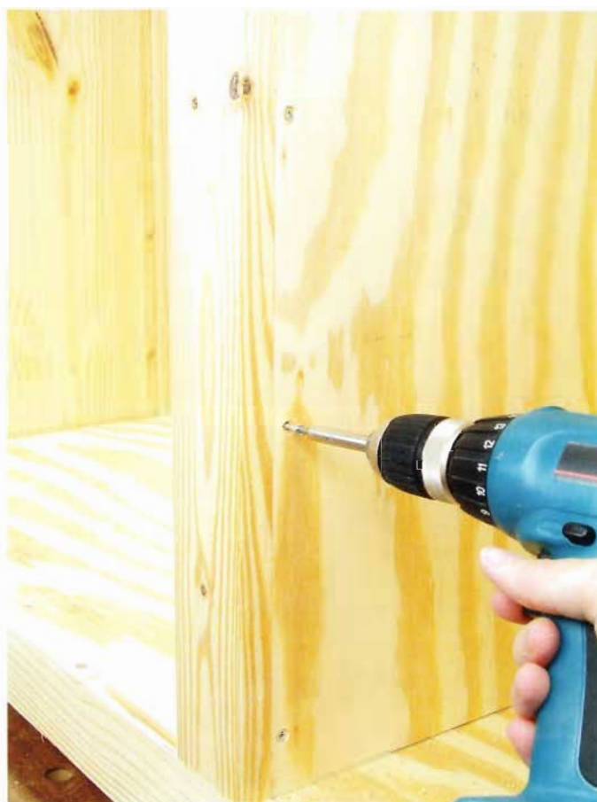
14 Drill holes in the interior panels. Using screws, install the interior panels against the cleats.
