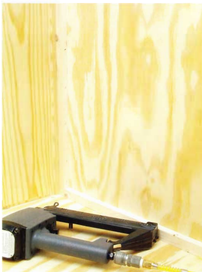
13 Using staples or screws, install the interior panel cleats for both interior panels.
