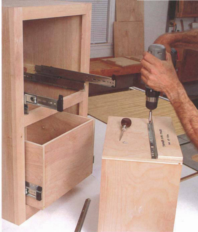
PHOTO E: After installing the sliding rail assemblies to the case, attach the quick-disconnect rails to the drawer box sides. A plywood spacer quickly and accurately positions the rails.
