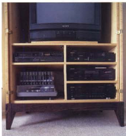
A center divider supports the weight of the television and partitions the lower cabinet for stereo components and a VCR.
