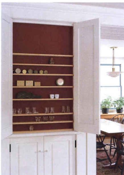
Extra storage always helps. One of the cabinets was designed to enclose the flues for the furnace and the woodstove, but it also provides room for storage.
