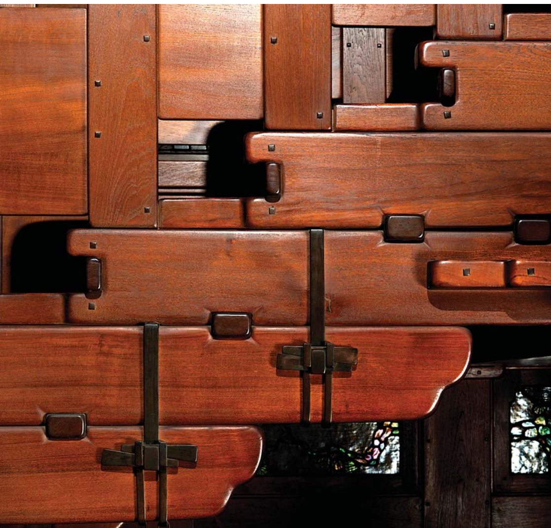
ABOVE Straightforward details, such as rectangular pegs in the newel posts and round pegs in the treads, create interest. Detail, stairs, William T. Bolton house.
