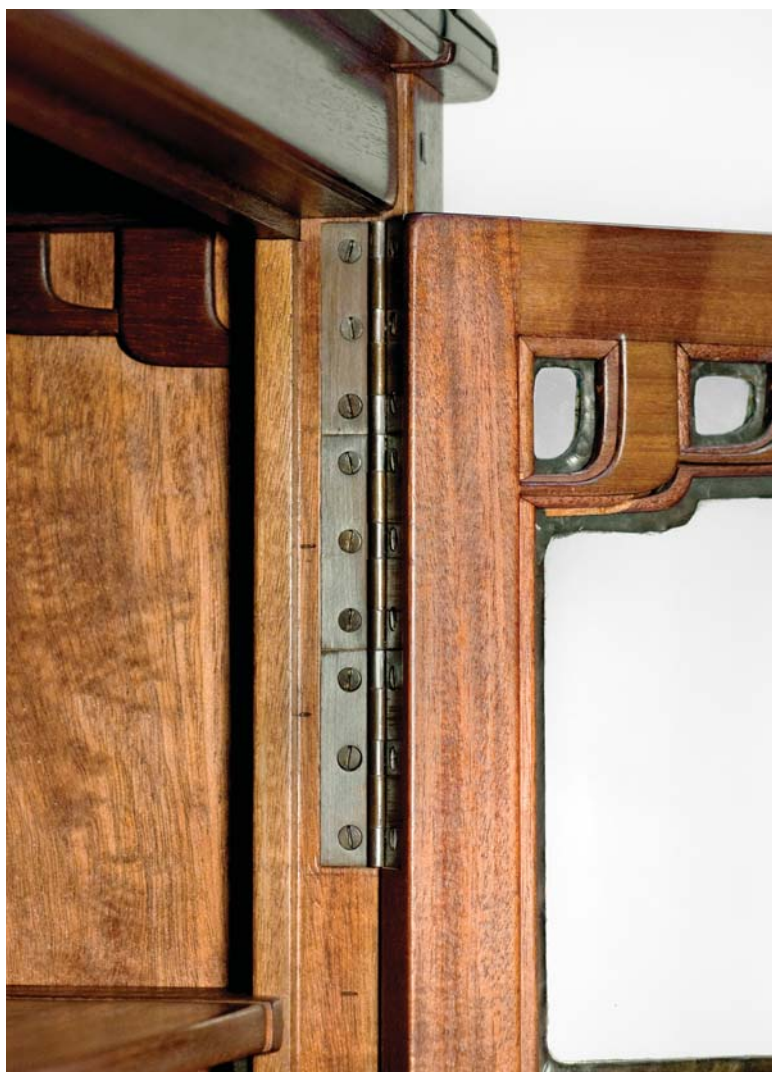
RIGHT A study of construction secrets: glass installation, shelf breadboards and supports, hinges, and brackets on the interior of the piece. Detail, living room bookcase, Robert R. Blacker house.
