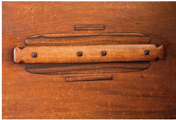
This drawer demonstrates the wonderful variety achieved with relatively simple building blocks. A similar flange, behind the pull, was used in the Blacker house entry hall. Detail, living-room bookcase, William R. Thorsen house.
