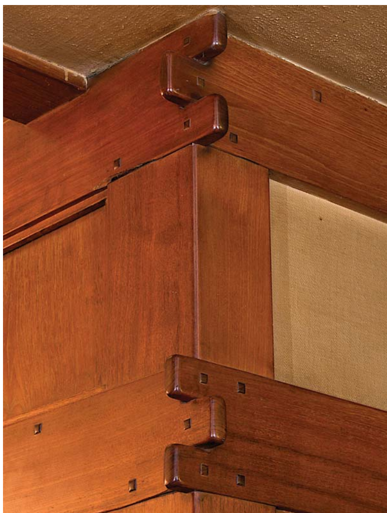
TOP Each finger in this joint is a different width, creating additional interest in a beautiful feature. Detail, hall table, David B. Gamble house.
