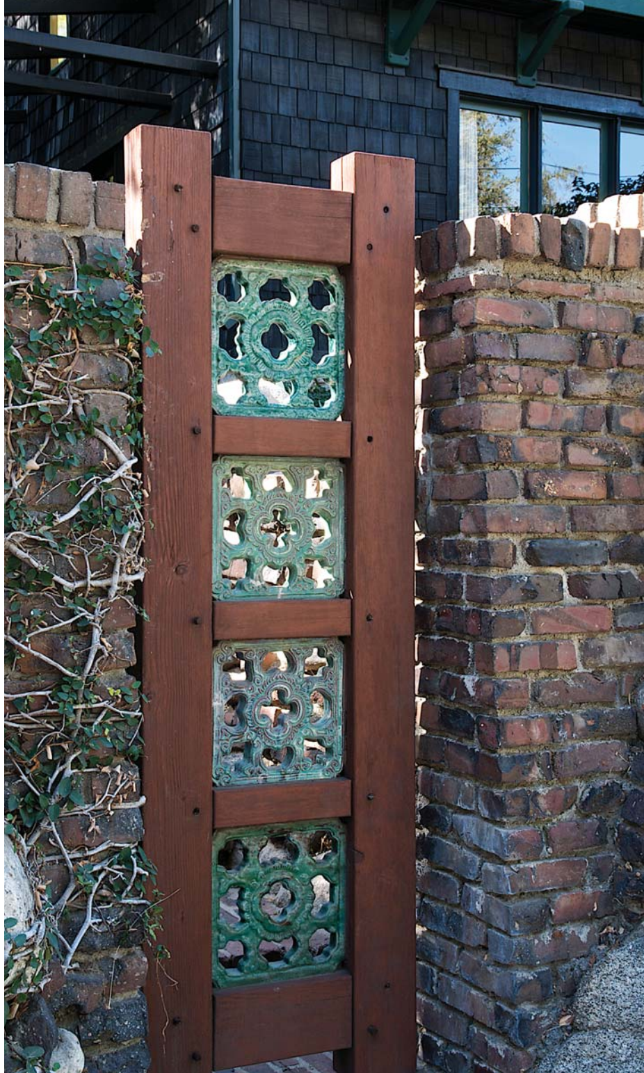
The Van Rossem house (the first of three) is the site of an amazing clinker brick wall. This gate, with Chinese tiles, clearly shows the Asian influence on the Greenses' work. Detail, wall and north façade, Josephine Van Rossem house #1, Pasadena, 1903.
