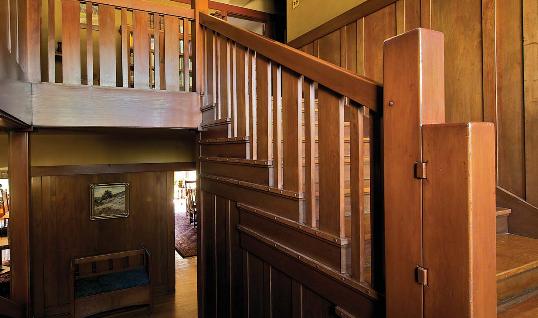
ABOVE Straightforward details, such as rectangular pegs in the newel posts and round pegs in the treads, create interest. Detail, stairs, William T. Bolton house.
