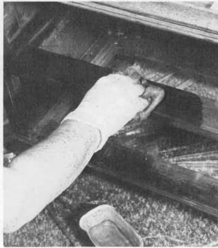
A test patch of the finish indicated that the original stain was in fair condition, so we removed only the old finish, using Formby's Refinisher and steel wool pads.
