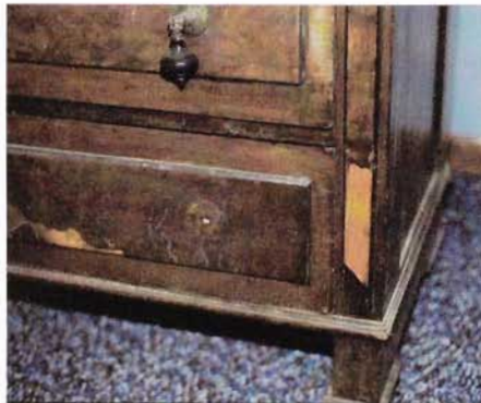
3 One of the most important problems that this dresser has is the missing veneer strips along the sides of the drawer openings. We must find replacement veneer that is of the same kind of wood.
