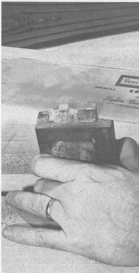
4 Now the broken tenon is sawed off flush with the end of the rail.
