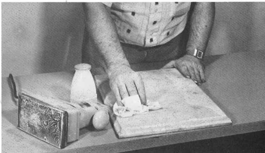
Wipe the marble clean occasionally to see how you are progressing. The process may take half an hour or more, depending on the depths of the pits and scratches. When the marble is smooth and beautiful, wash off all the white paste, allow the stone to dry, and apply a good marble polish.
