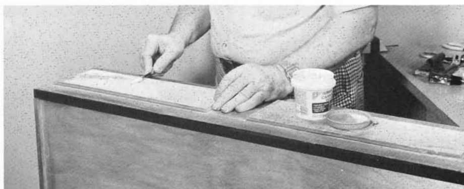
To cover a few chisel marks and some old indentations on the surface, use a spatula to wipe a wood filler across the surface. Don't build up the old surface; just fill the dents.
