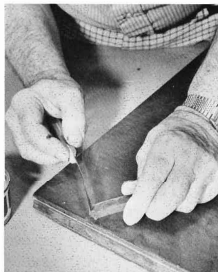
Apply the hot spatula blade to the stick of shellac as you hold it over the repair. Allow the shellac to drip into the repair or lift some of the soft shellac with the blade.
