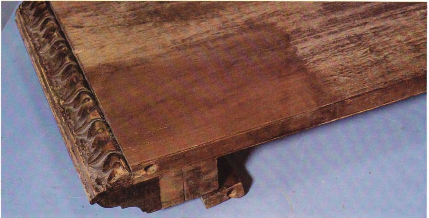
11 The patch is difficult to see. To hide it further, a second light application of stain might be necessary after the first has dried. Finish by lightly sanding, then applying varnish or lacquer.
