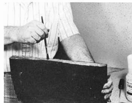
The oak chair was reglued after the seat broke, and the repair didn't hold. Apply warm vinegar and water to soften the old glue.
