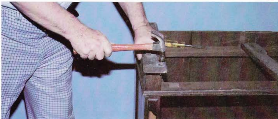
7 The old square nails have been left in and are now hammered into place as the base plate is glued back on the dresser.
