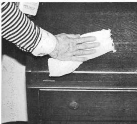
Old furniture has layers of wax, grit and grime, and the first step in restoring it is to clean the finish.
