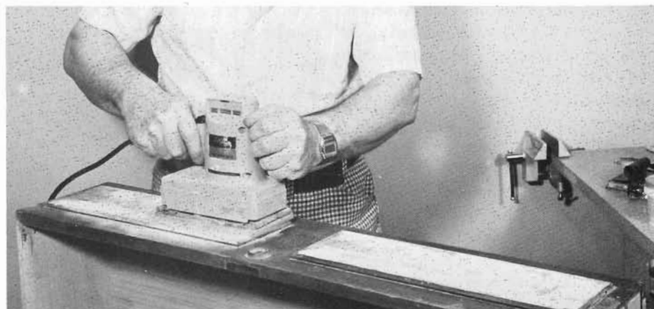
After the filler has dried, sand again to make sure the surface is perfectly smooth.
