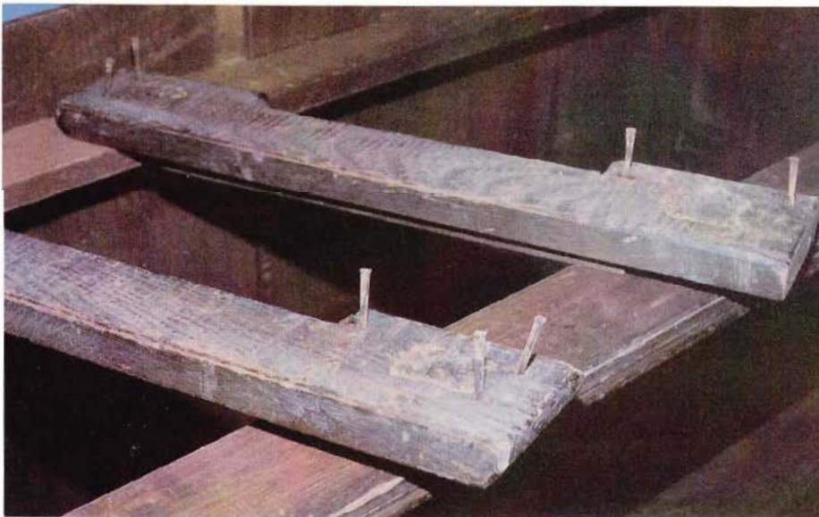
6 The base plates look bad. Should we replace them? We decide that the wood is sound, and only the appearance is bad. It is important in restoration to retain as much of the original wood as possible, hence the decision to sand and replace these base plates. Note the old square nails, a good clue to age. These nails were not used much after 1890, and not at all after 1895.
