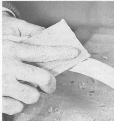
6 After the glue had dried, the repaired arm is sanded smooth. Wood filler is used to fill the edges of the repair area.
