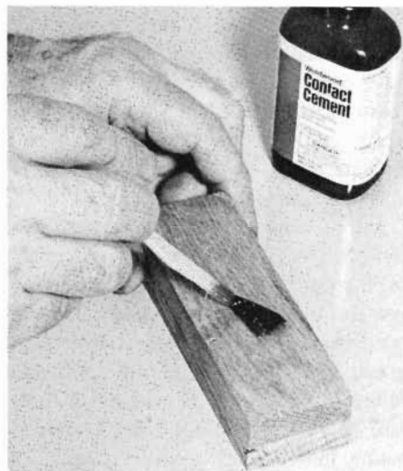
Coat the wood block with contact cement; allow to dry. Repeat on one side of the padding.
