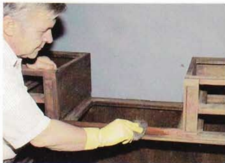
1 Using a furniture refinisher (Formby, Hope, Squaw Alley brands) and 0000 steel wool, we strip away the old finish, leaving the original stain and the wood's patina.
