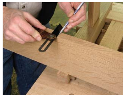
An adjustable bevel transfers the layout lines for the angled mortise from the top of the arm to the bottom.
