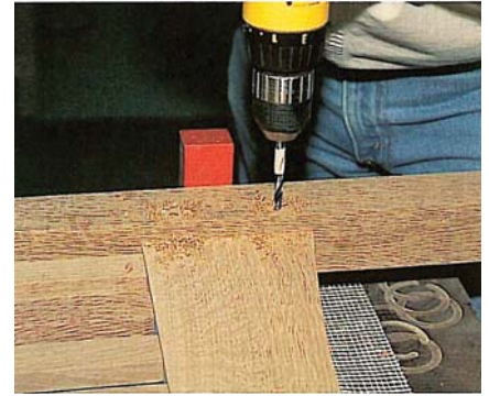
When drilling the peg holes, a piece of tape on the drill bit provides an inexpensive depth gauge.
