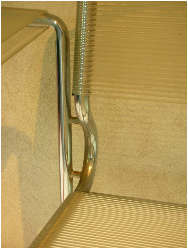
Figure 7.22 Elastomeric PVC tubing in the Spaghetti chair. Designed by Giandomenico Belotti (1979–1983), for Alias SpA. 32¾ inches high; 15 7/8 inches wide; 20 1/8 inches deep; 18¼ inches seat height (83.2 high; 40.3 wide; 51.1 cm deep; seat height 46.4 cm). Photography by Jim Postell, 1990.
