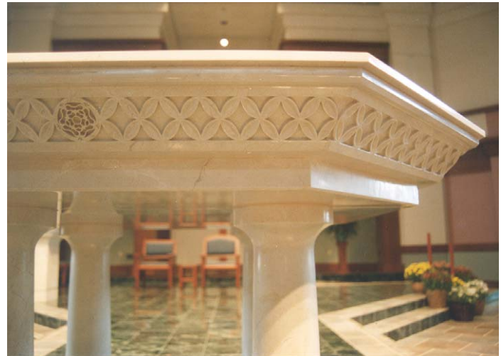
Figure 8.11 Milled relief design cut into a marble mensa, made using a digital, three-axis CNC. Photography by Jim Postell, 2002.
