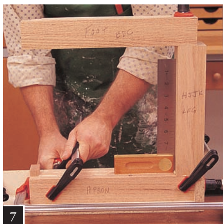
7 Leg/foot assembly HJJK/BDC is glued to apron BDC. (Note the use of a square. This tool will be used throughout all of these projects. It is very important that all joints be square. This will make later assemblies that much easier to keep square.)
