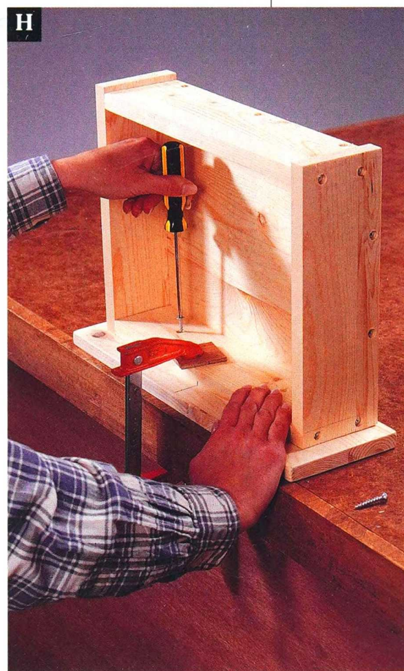
Align the drawer front, and attach the pieces by driving screws through the drawer end.
