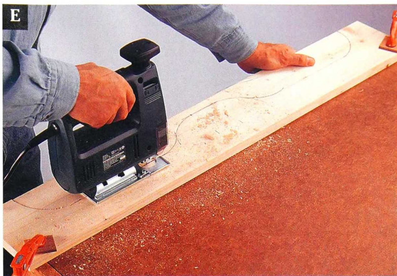
E Lay out the decorative cutout at the bottom of the front skirt board, using a compass to make the curves. Then, cut with a jig saw.
