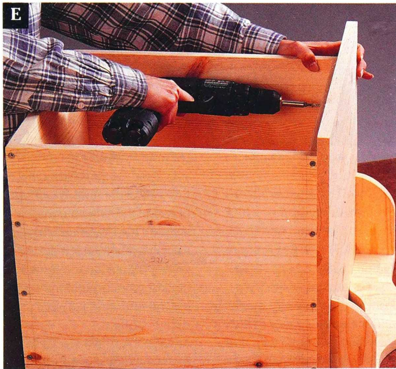
E Attach the top assembly to the top shelf with glue and screws.
