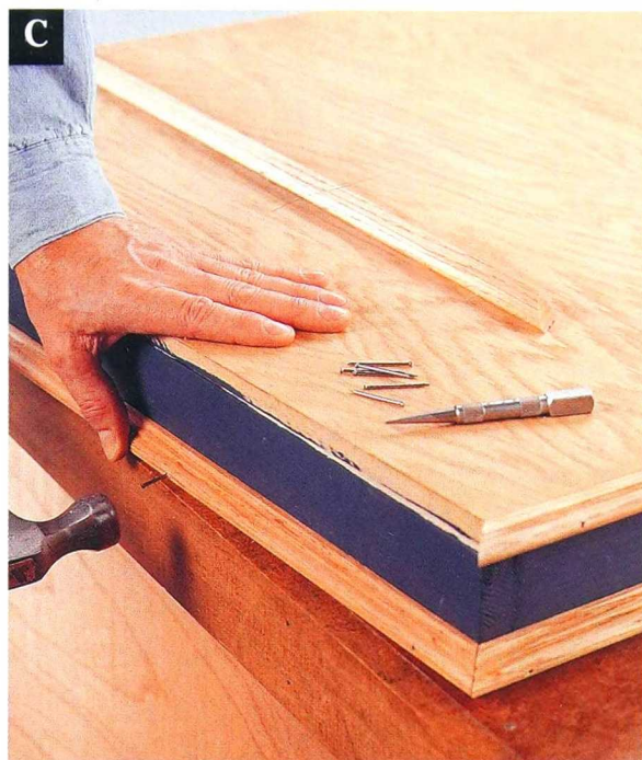
C Glue and nail oak trim around the tabletop and apron, making mitered joints at the corners.
