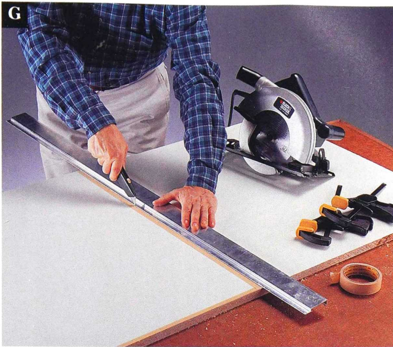
Score the cutting lines on the melamine with a sharp utility knife to prevent chipping.
