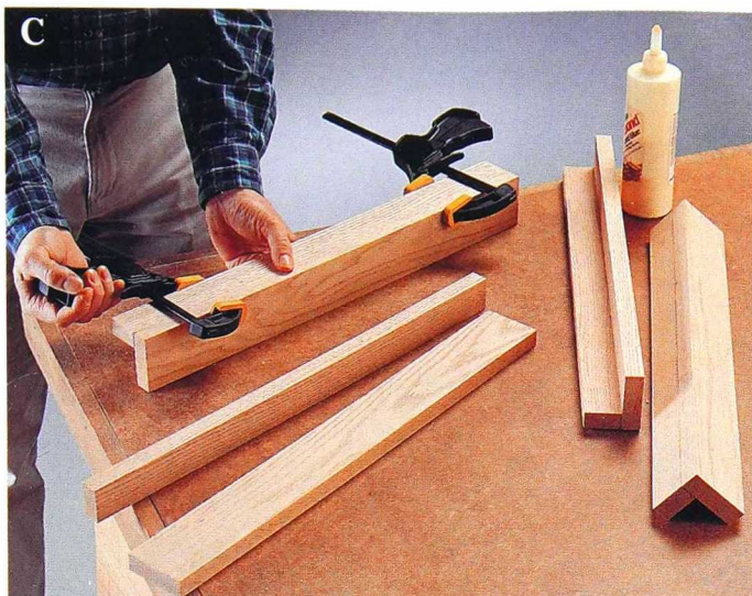
Join the wide and narrow leg pieces with glue; when this is done carefully no nails or screws are required.
