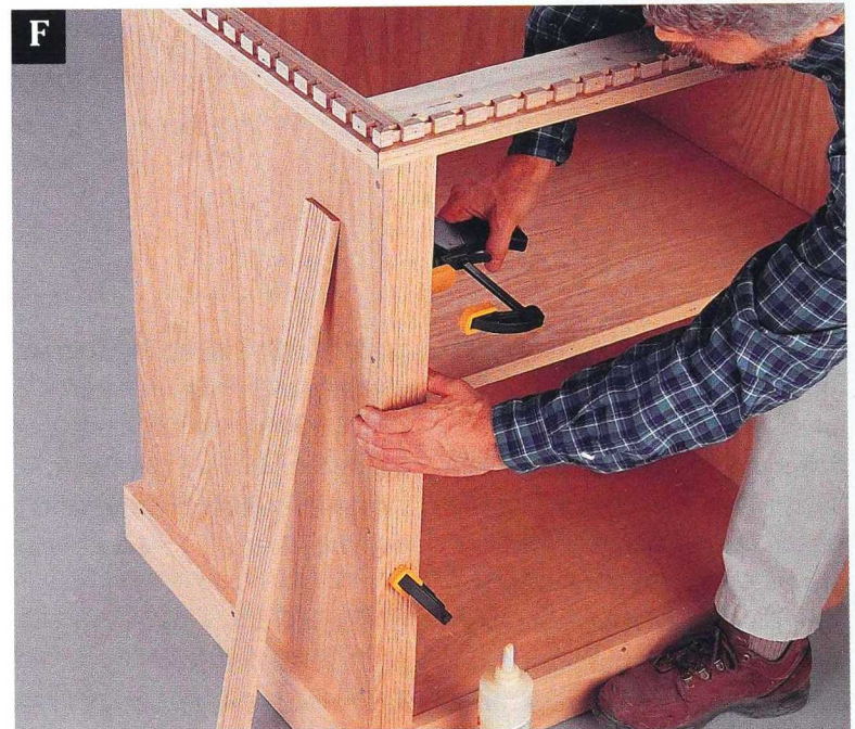
Clamp the corner molding in place to ensure a tight bond with the posts as the glue dries.
