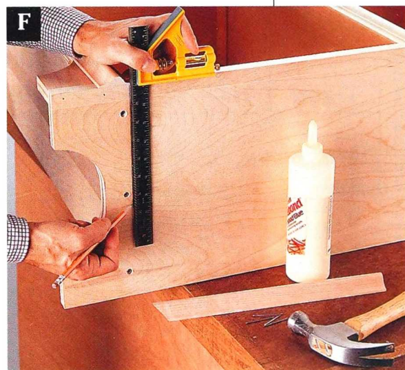
F Using a combination square, draw lines on the sides, aligned with the top of the bottom facing.
