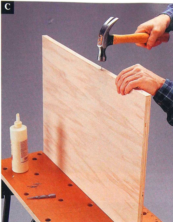
Use glue and brads to attach shelf nosing to the front edge of the shelf.
