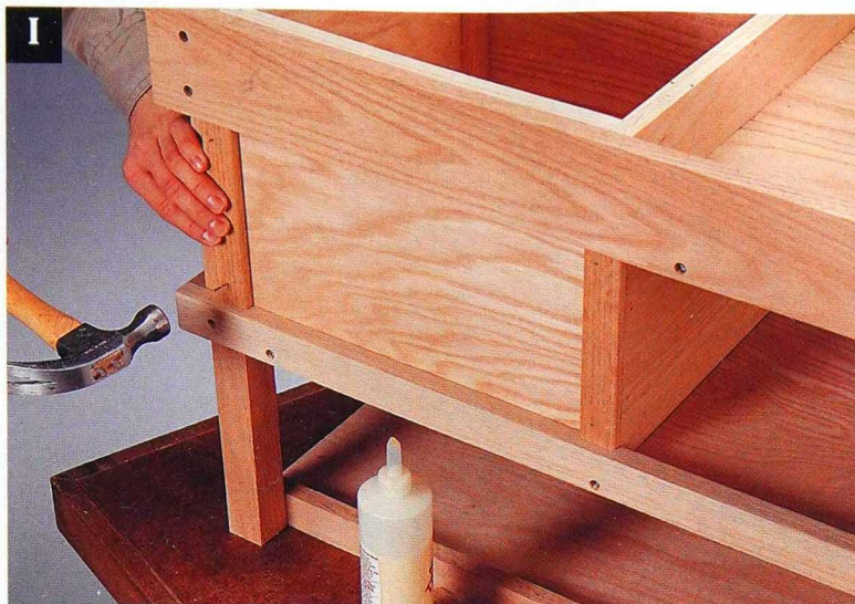
Attach strips of oak stop molding to cover the exposed plywood edges of the bins on the outside of the credenza.
