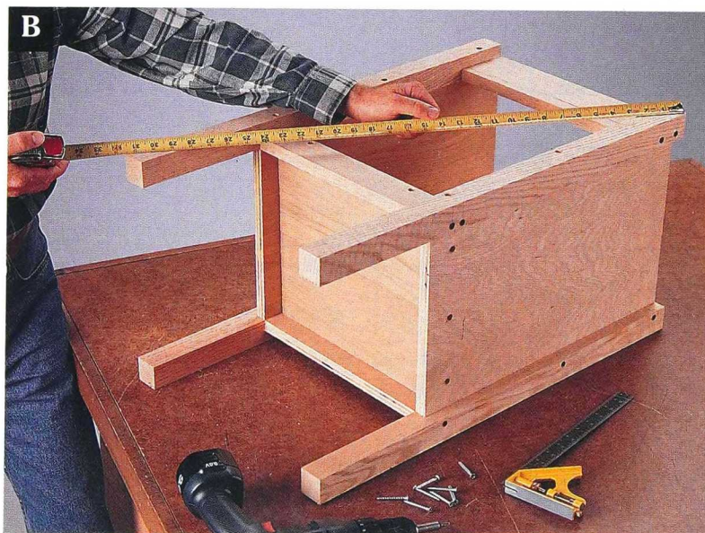
Measure from corner to corner to check for square. If the project isn't square, apply pressure to one side or the other until it is square.
