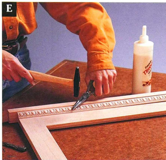
E Center egg-and-dart trim molding under the cap, and attach it with glue and brads.
