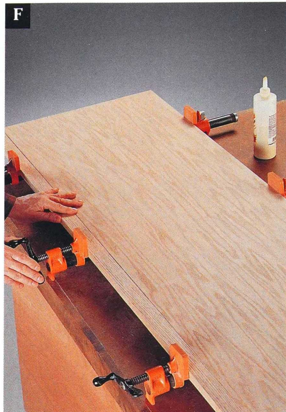
Glue the platform nosing to the platform and hold it in place with bar clamps.
