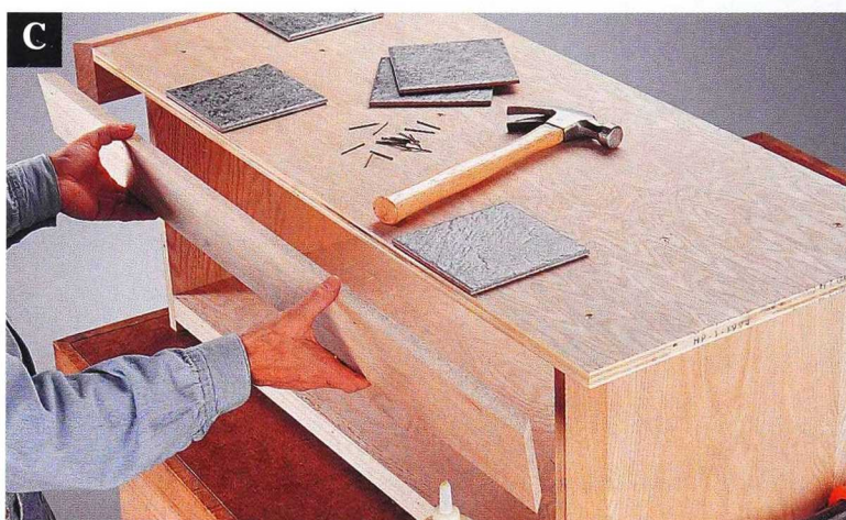
Miter-cut and attach one skirt board at a time to ensure a proper fit.
