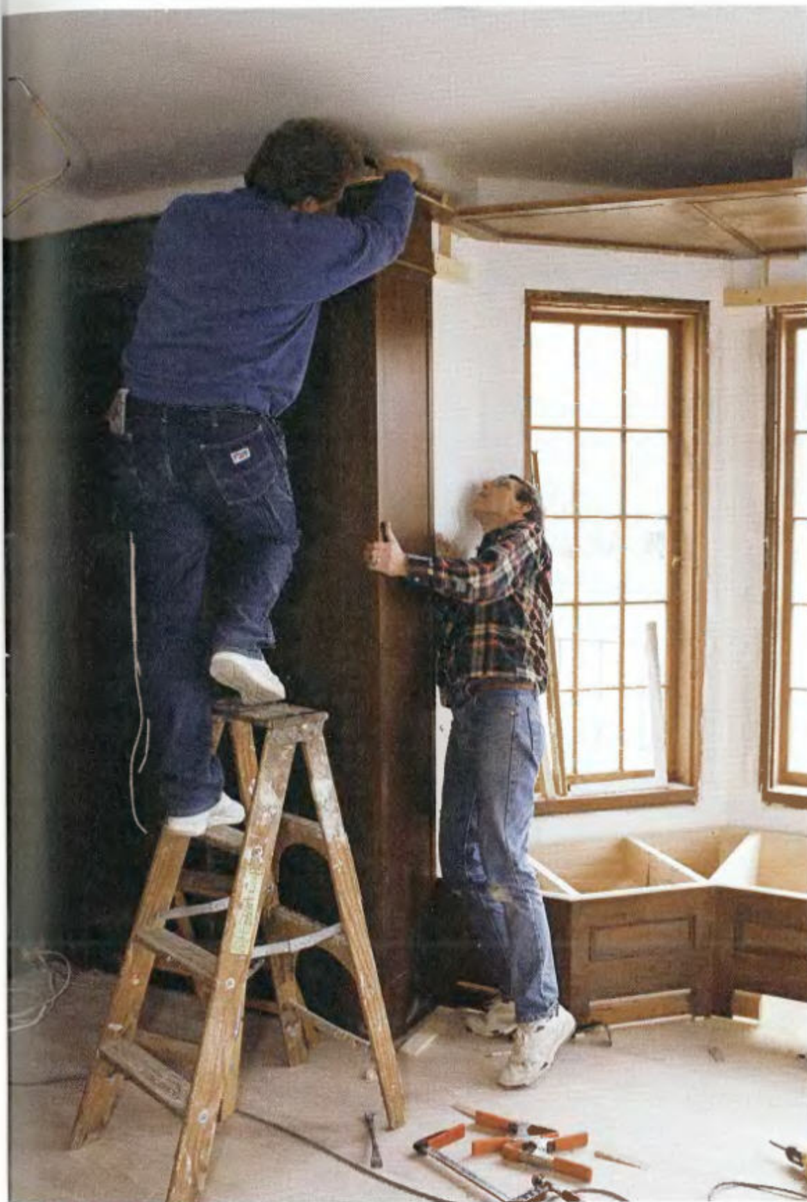
INSTALLING THE CASE WORK. Job-site conditions usually require shims to make cases level and plumb. The result is a beautiful library and plenty of sawdust back at the shop
