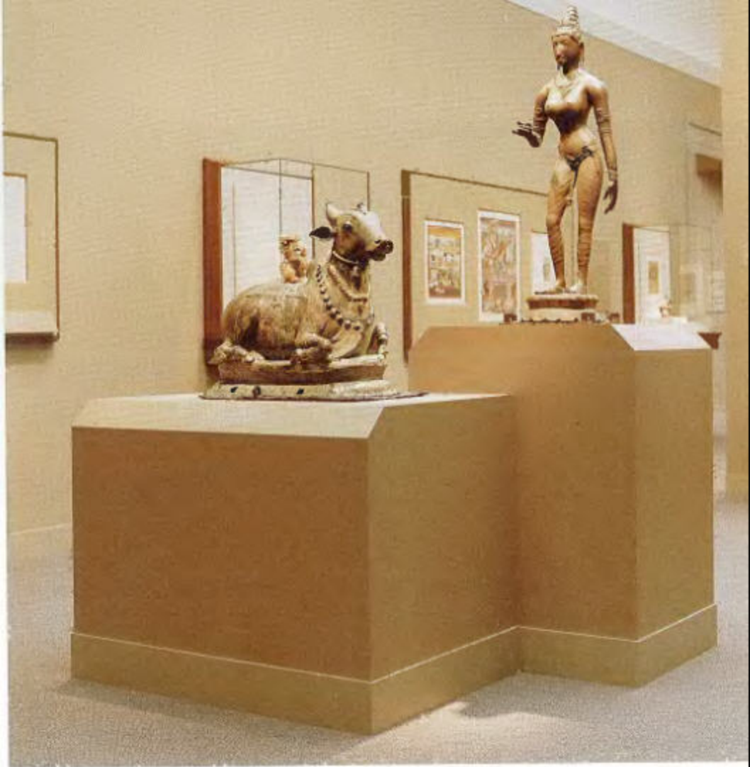
MUSEUM-QUALITY MDF. These display cases at the Freer Gallery of the Smithsonian Institution show off some of MDF's versatility. The case pictured above shows the crisp edge-holding ability of MDF in a painted piece. The case shown below makes use of walnut-veneered MDF with solid-wood moldings.
