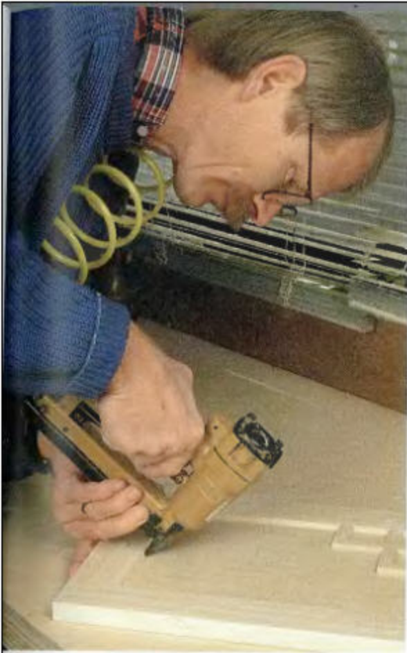
NAIL IN THE RAIL. The author shoots brads through the frame of the door to keep it from shrinking away from the panel, which could crack the paint and expose unfinished wood.
