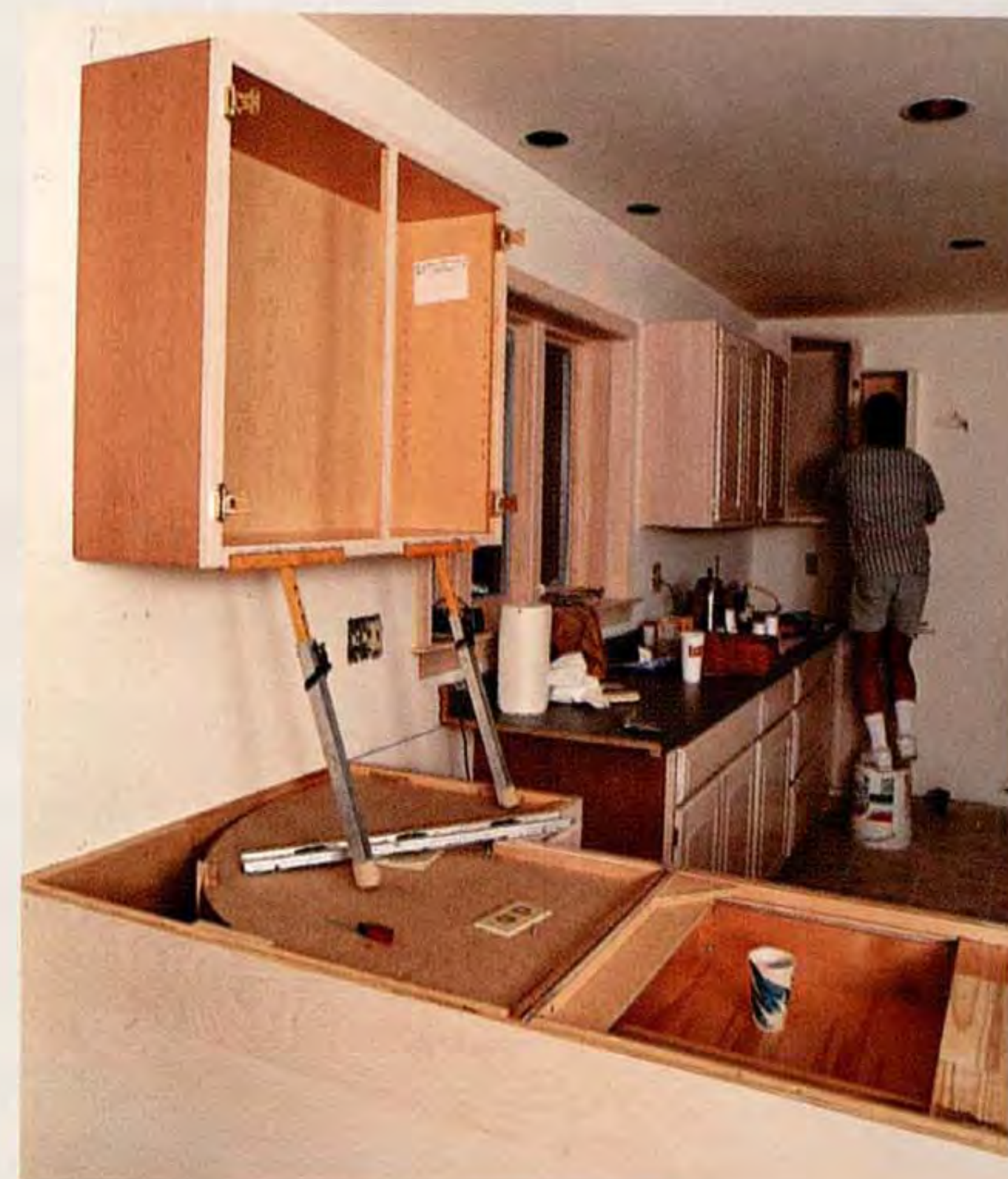
Cabinet jacks consist of square steel tubes that slide inside each other; a cabinet sits in cushioned angle iron.
