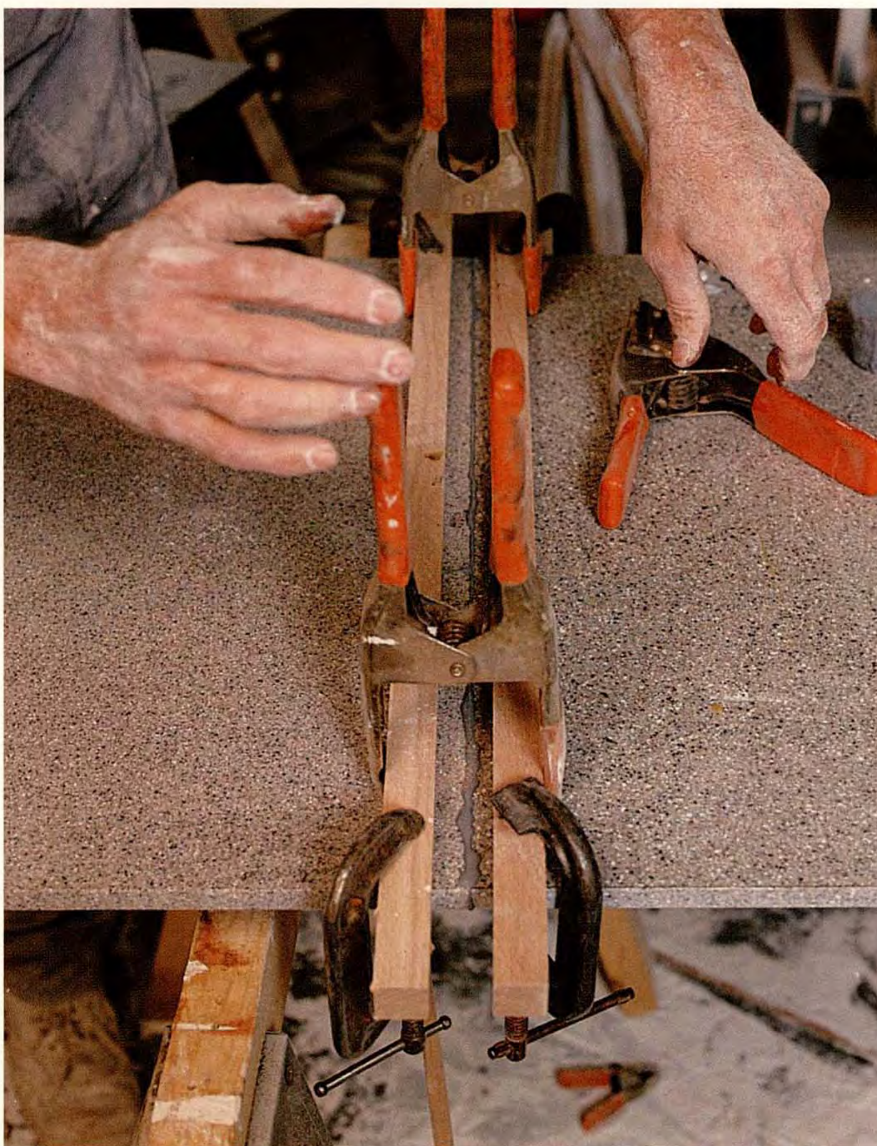
Fill, then clamp. During glue up, adjoining pieces are kept 1/8 in. apart while glue is drizzled into the gap. Then the pieces are put together, and spring clamps are applied on 3-in. centers to the 1x clamping blocks.
