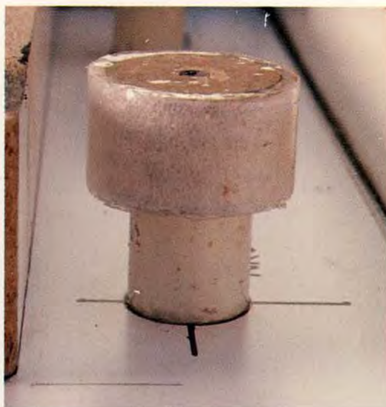
Faucet and air-gap knockouts are made with MDF disks, wrapped with sheet foam and packing tape and screwed down through a short length of 1½-in. PVC pipe.
