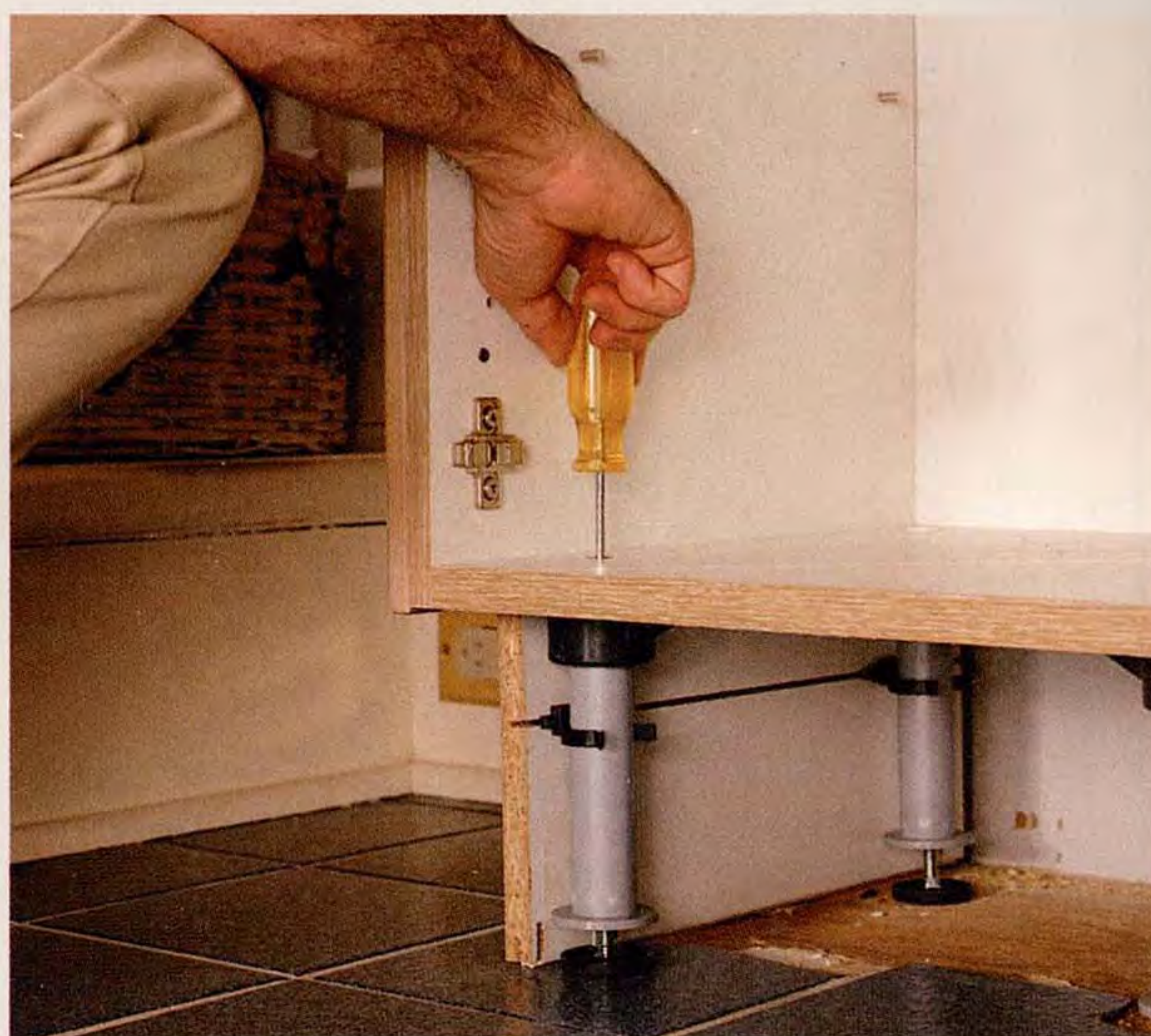
Adjusting the leg. You don't have to shim or scribe European cabinets because they rest on legs that are adjusted up or down with a screwdriver. The toe kick clips onto the legs; the clips are also adjustable.
