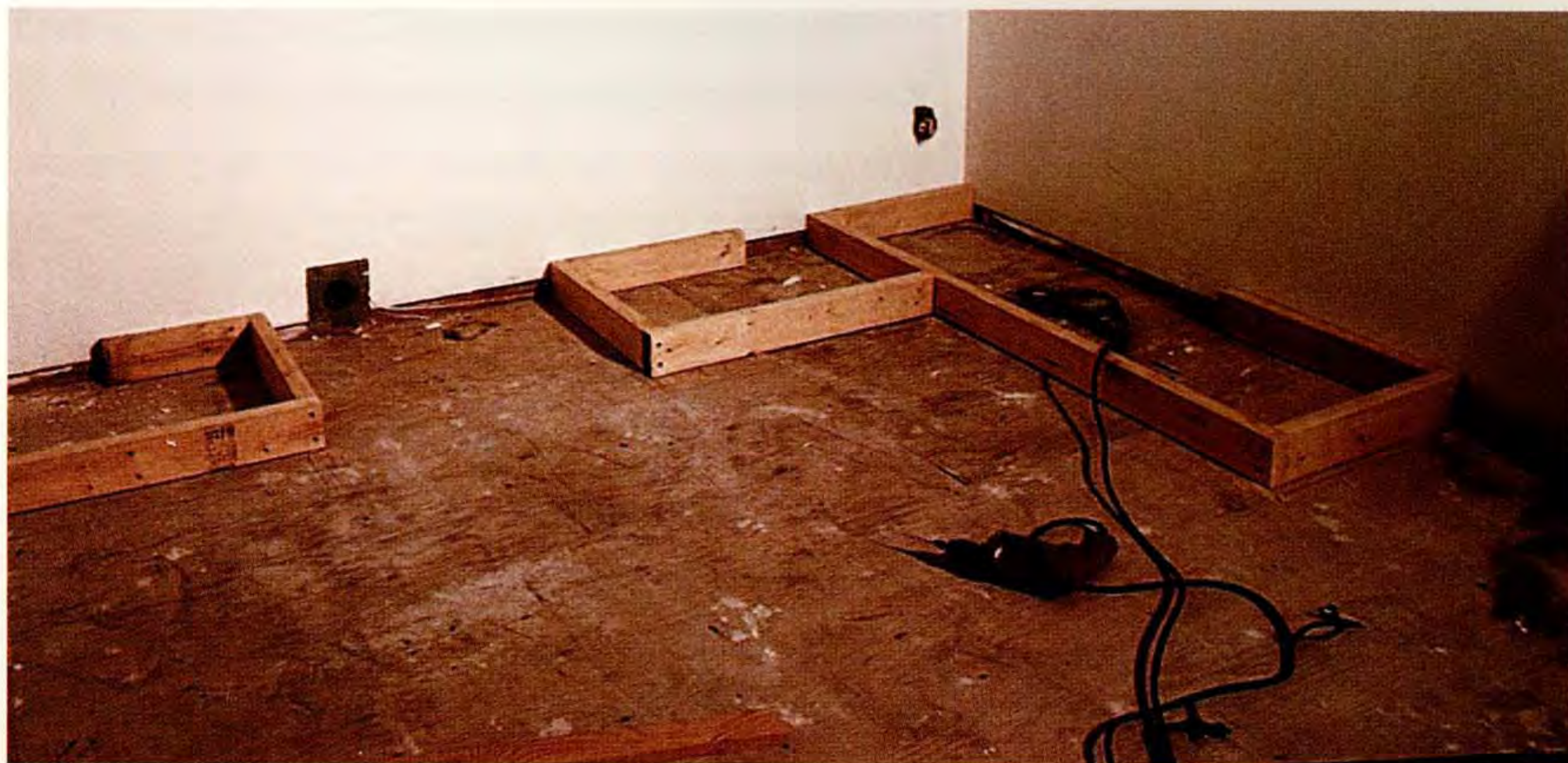
First the frame. The author assembled the base cabinets atop a frame of 2x4s toenailed to the wall and the subfloor.
