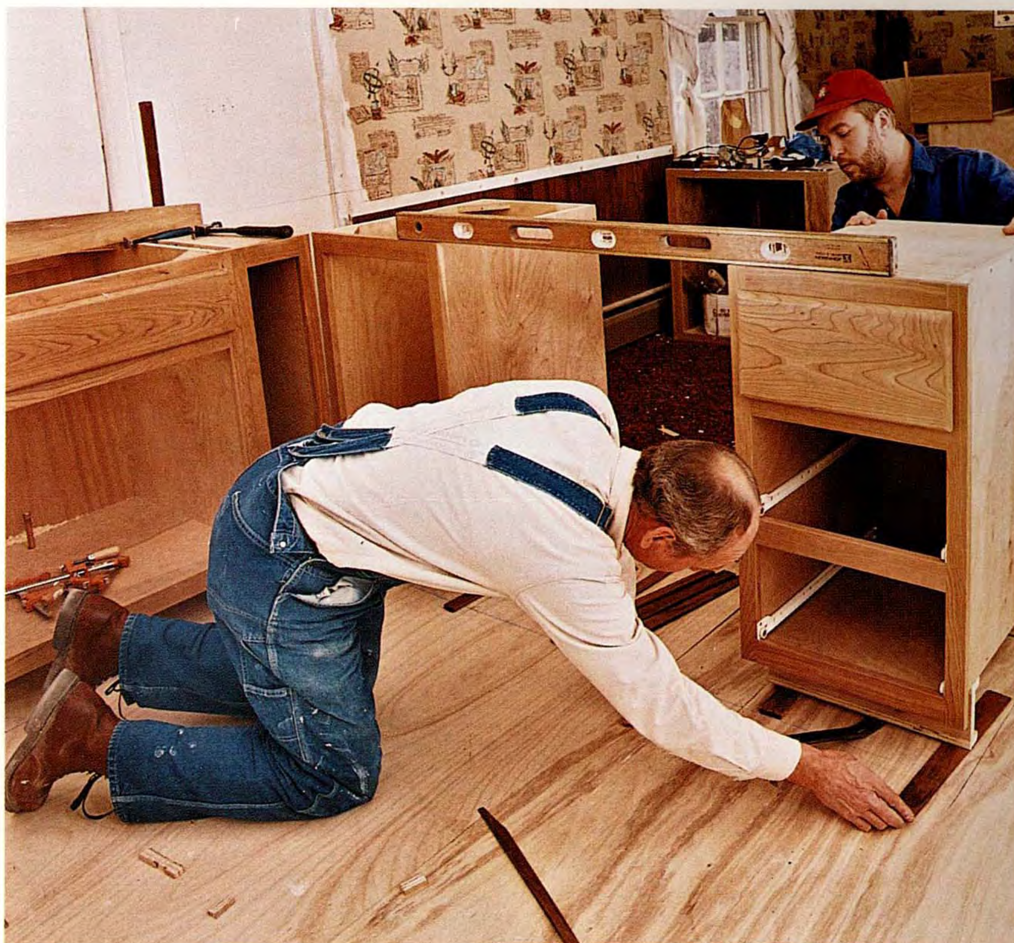
Shimming a cabinet. Shims are used to level a cabinet, but they also bring cabinets that sit in low spots of the floor up to the proper height. Here, the end cabinet of a peninsula is leveled.
