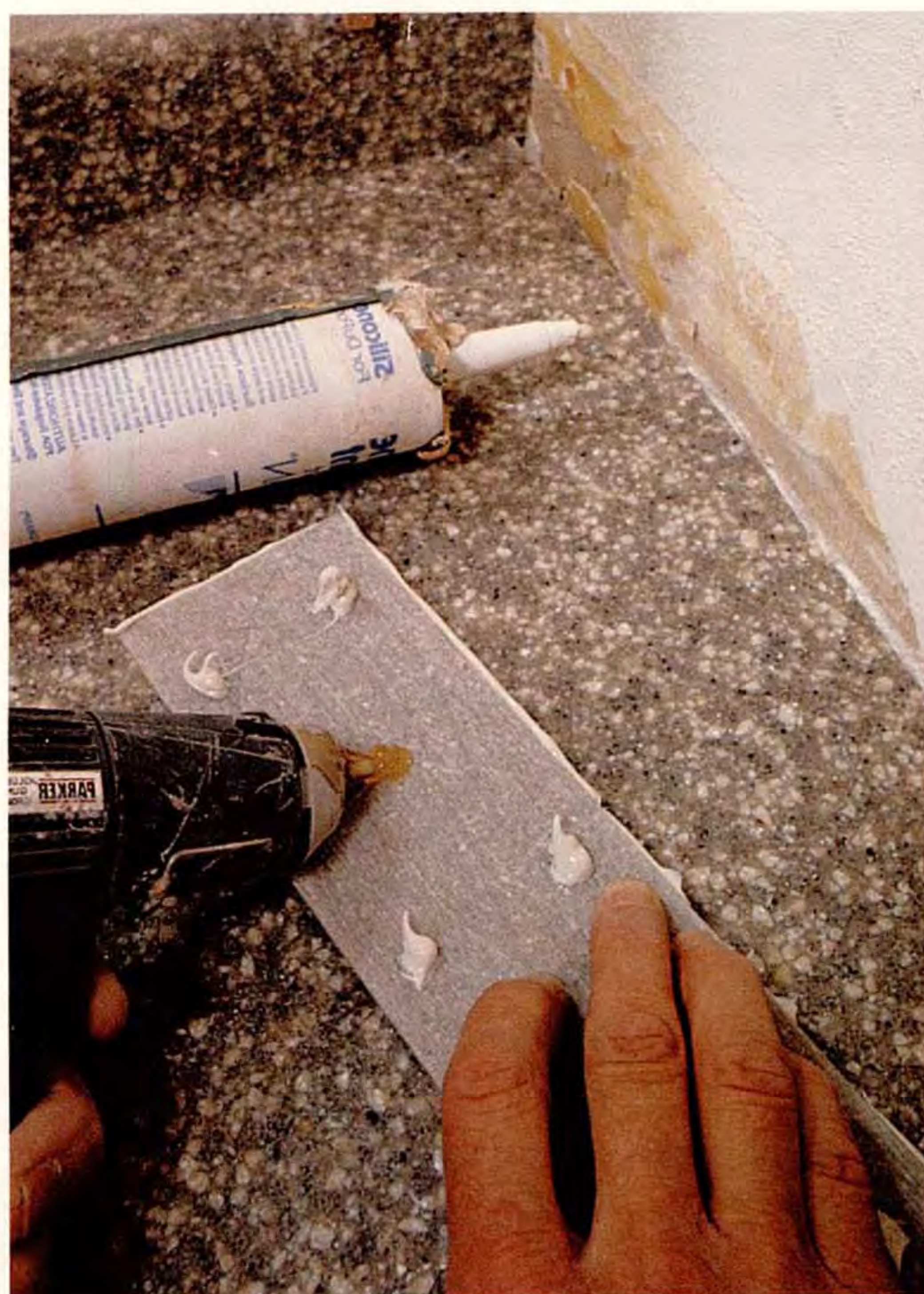
Splash. Counter backsplashes are attached to the wall with silicone caulk and hot-melt glue. The hot-melt glue holds the backsplash in place while the caulk sets up.
