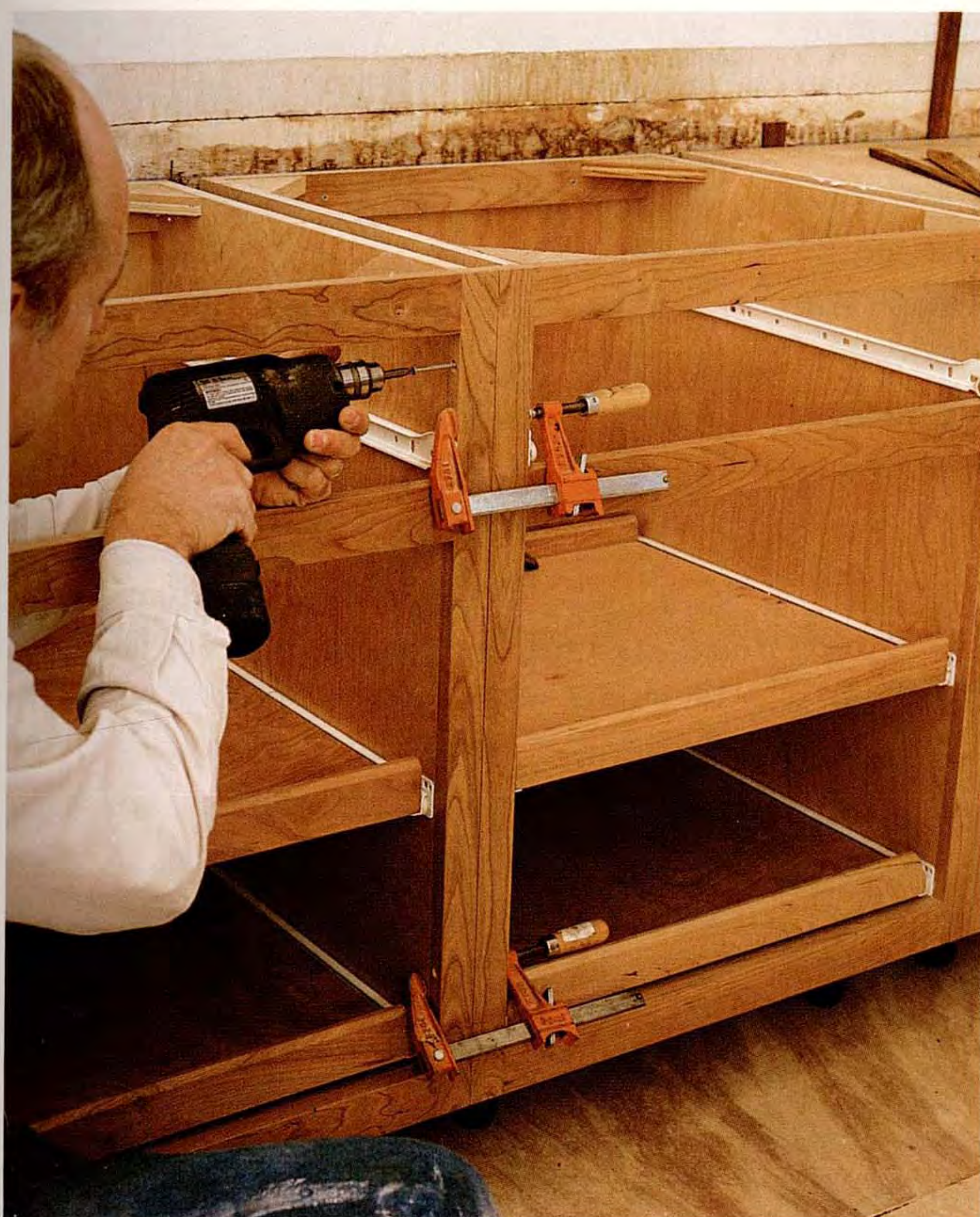
Joining cabinets. Cabinet stiles are clamped flush and joined with wood screws before the cabinets are installed. Two wood screws hold the cabinets together, one near each hinge.
