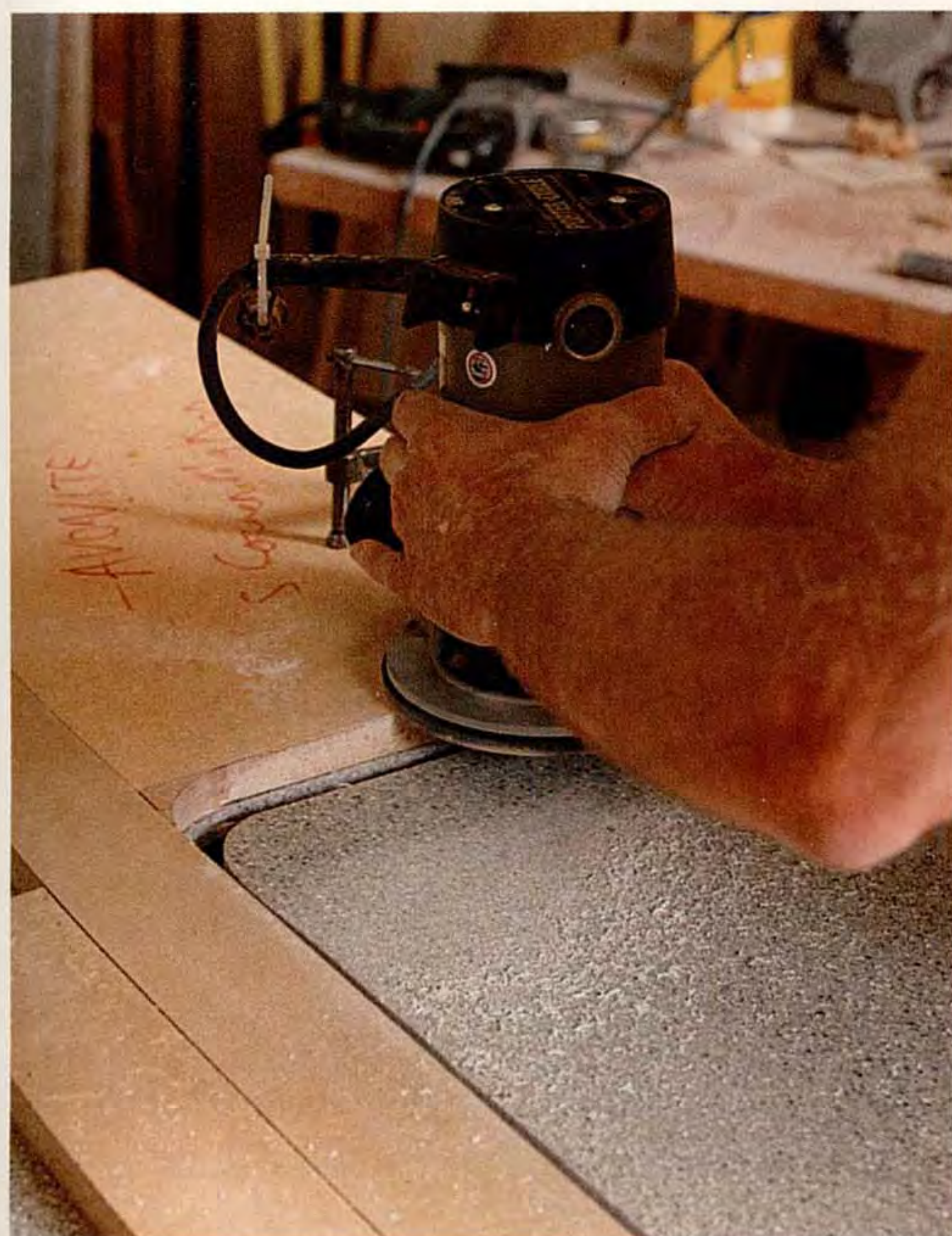
Cutting guide. Inside corners have to be radiused to reduce stress. This MDF cutting guide has a radiused wood insert at its corner.
