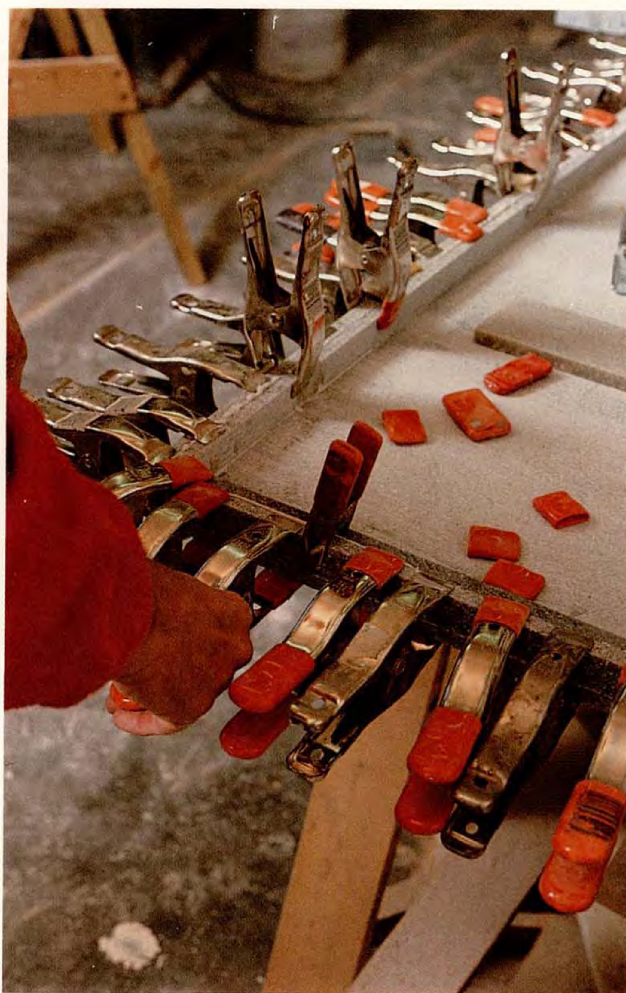
Clampfest. Built-up edges, or nosings, are formed out of two strips of Avonite. Here, a vertical strip is clamped to the counter's edge. Then a second strip is glued to its back.
