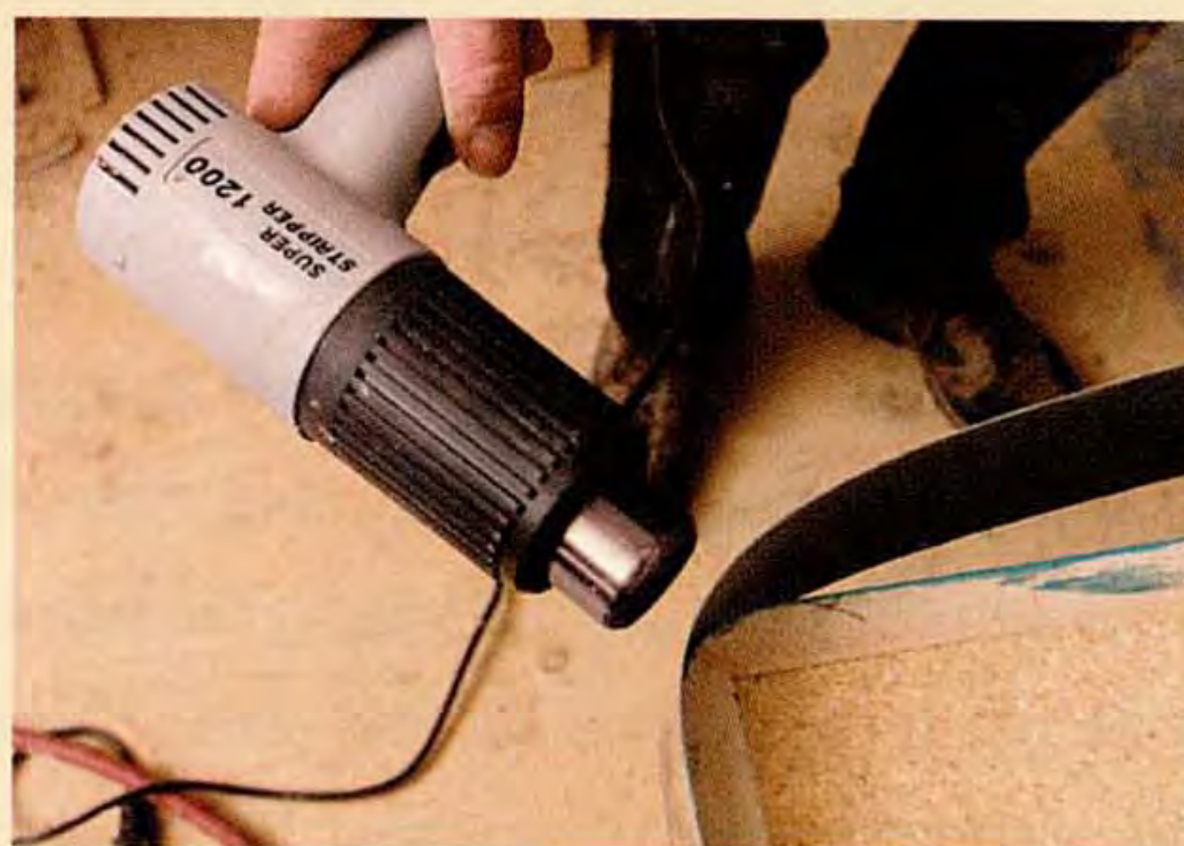
3. Heat laminate to make it flexible.
