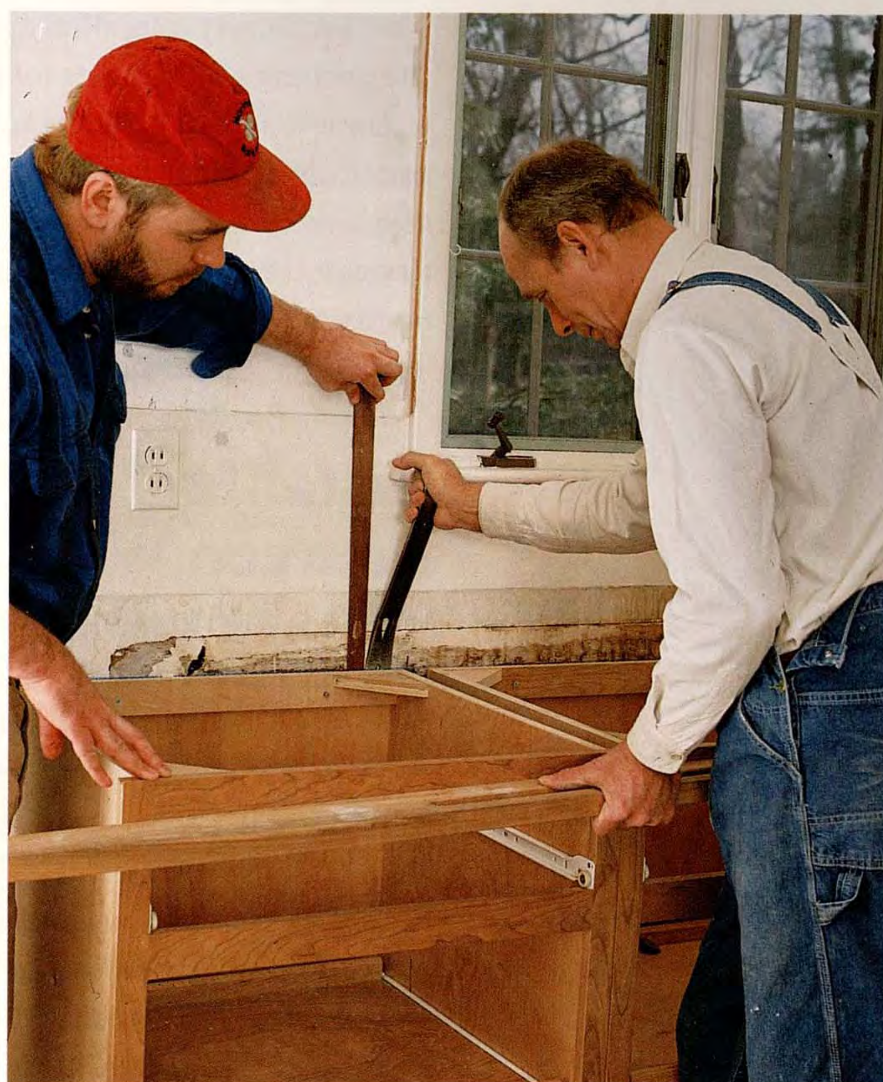
Aligning cabinets. A straightedge placed along a run of cabinets shows which cabinets must move in or out. Here, a cabinet is pried away from the wall and shimmed out.
