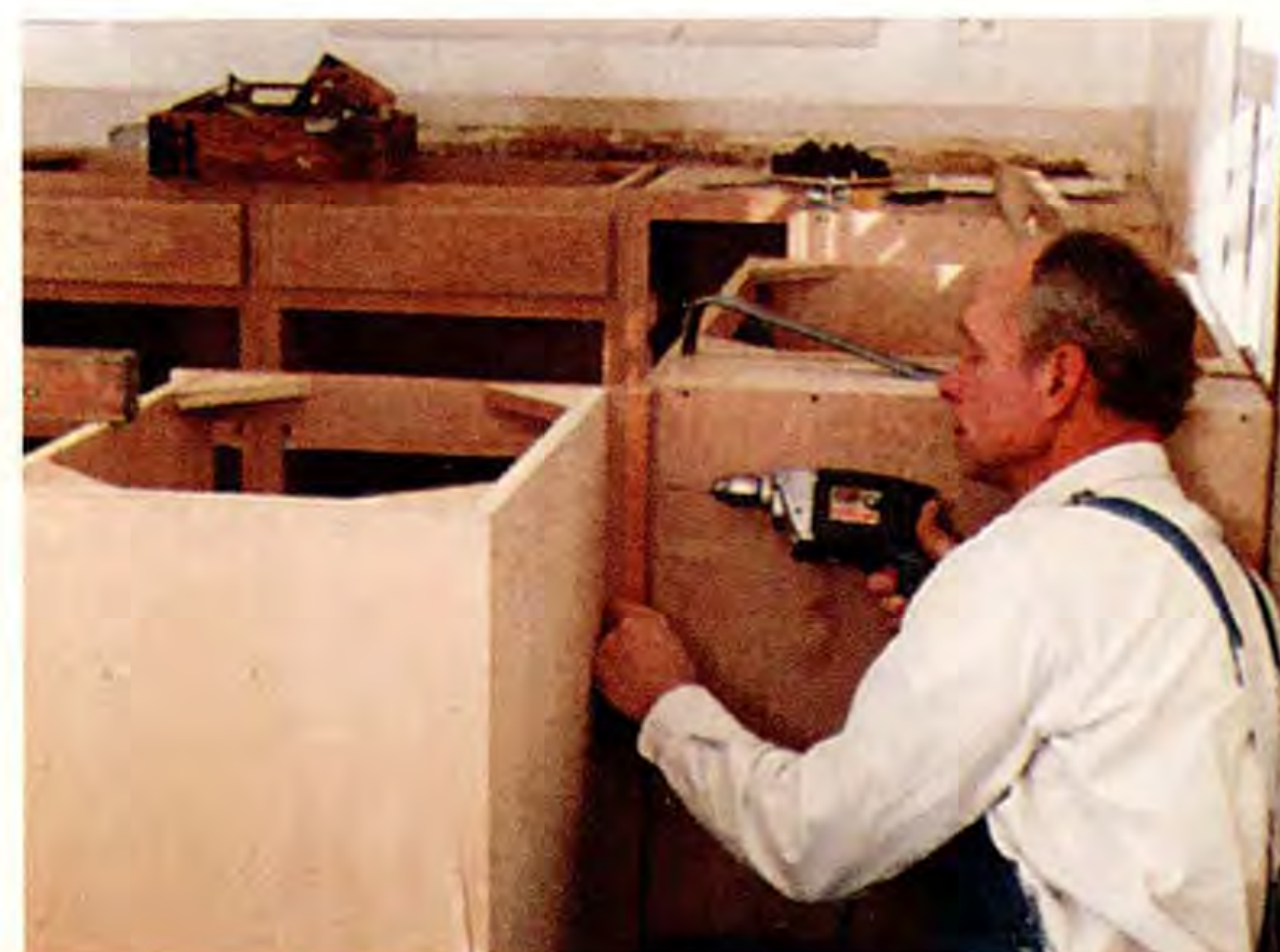
Fastening a backer strip. This strip of wood acts as a spacer to hold the corner cabinets far enough apart so that their drawers don't bump into each other.
