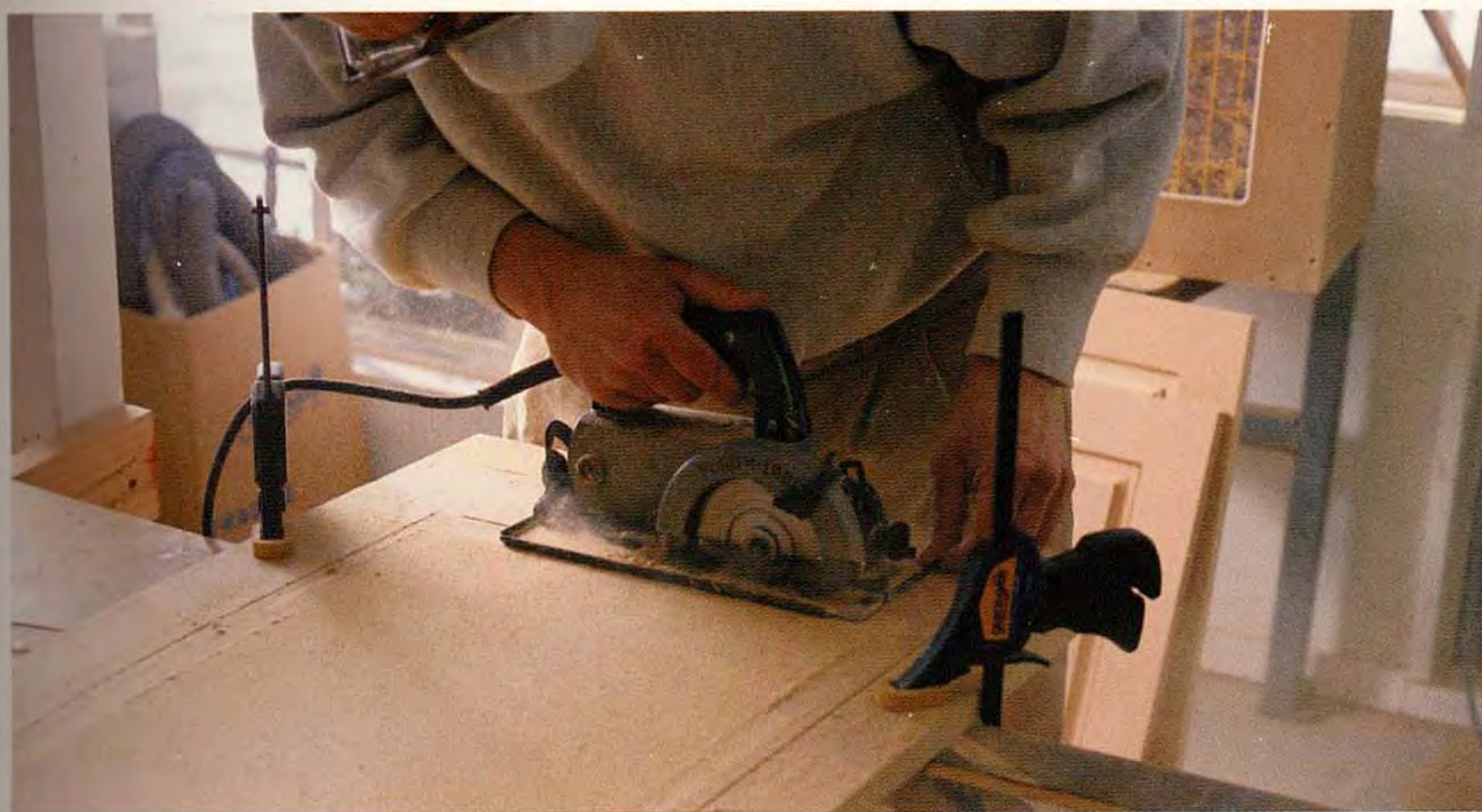
One-piece face frame cut from MDF. To create a decorative end panel, the author makes a face frame by cutting a rectangle from a piece of medium-density fiberboard.
