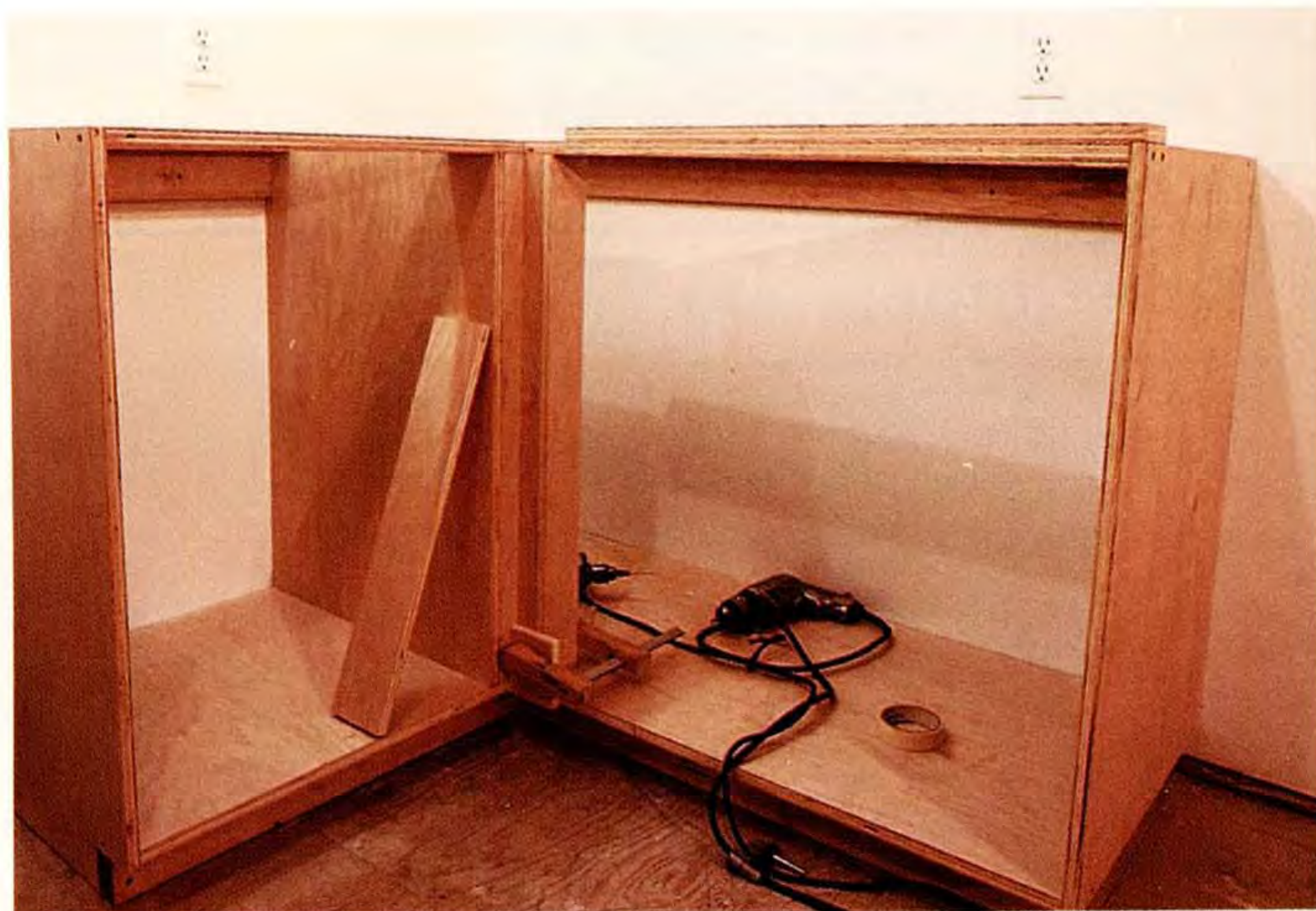
Inside corner. A built-up post made of three strips of plywood serves as an anchor for the cabinet-door hinges. The post is secured at the top by screws through the stretchers and at the other end by a couple of finish nails into the cabinet bottom.
