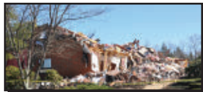
Sunco's old headquarters facility collapsed just over a year and a half ago under the weight of snow accumulation.
