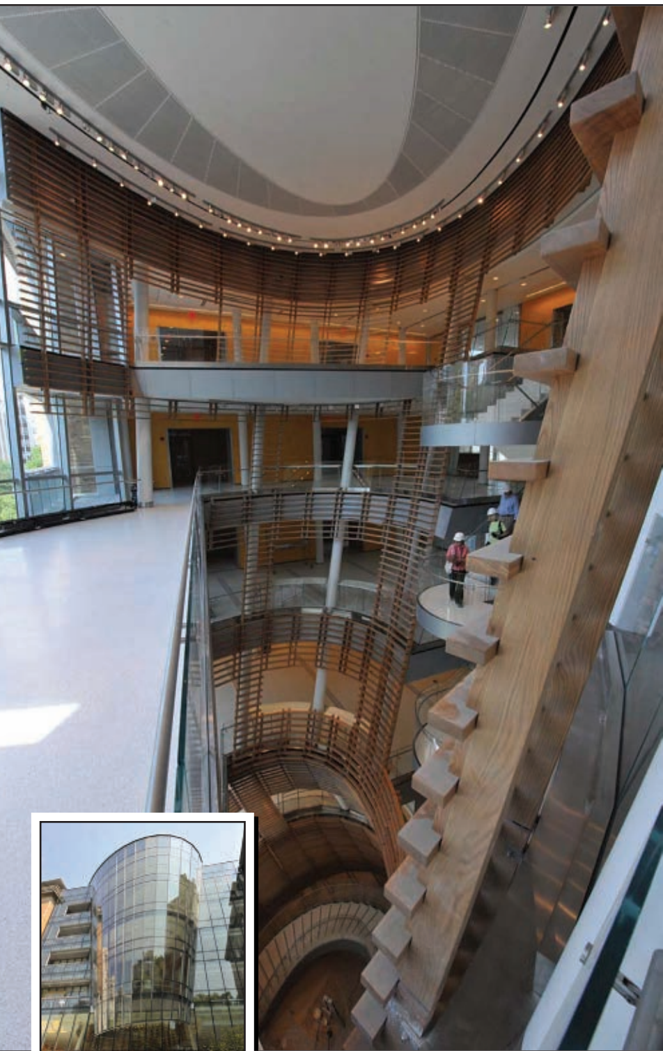
Eight-level Roosevelt University project features a metal structure with wood ribs that curves around an atrium.
