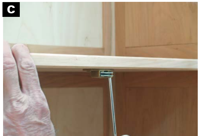
INSTALL A MAGNETIC CATCH under the fixed shelf to retain the doors in place when closed.
