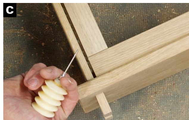
USE A SQUEEZE BOTTLE TO INJECT GLUE between the cabinet top and the top edge of the front stretcher to secure the front panel.
