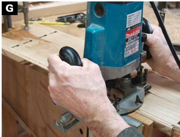
ROUT THE GROOVE FOR THE BACK. Set the router fence so that the cut is \frac{9}{16} in. from the edge of the stock.
