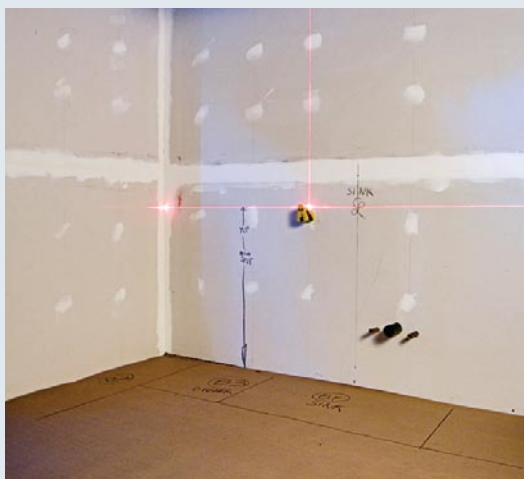
An inexpensive, self-leveling laser level—held to the wall with double-stick tape—shoots a line along the surface to create a reference line.
