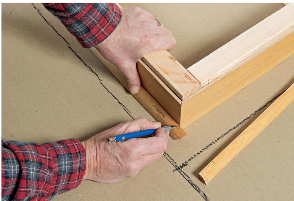
Holding the shoe molding in place, I mark the location of the corner miter cut.
