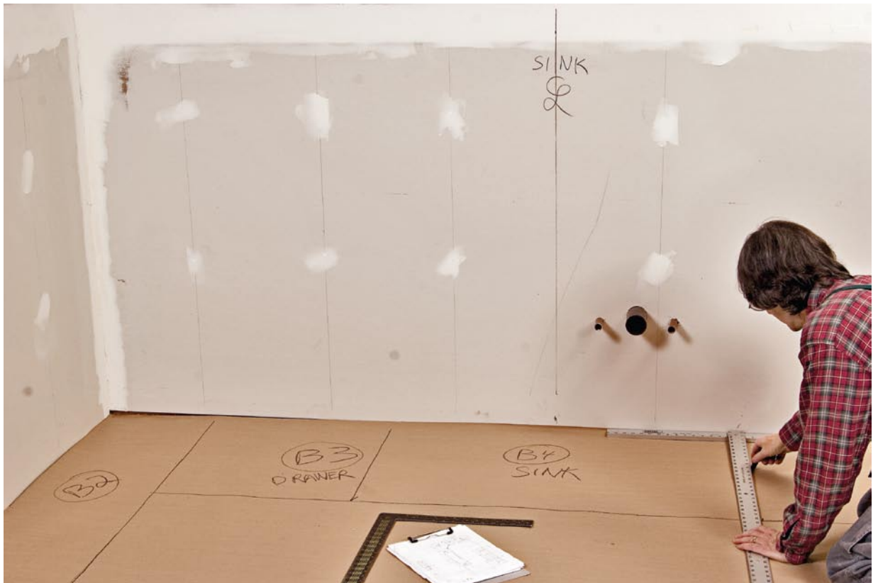
After laying down sheets of building paper, I lay out the kitchen cabinets full scale on site.
