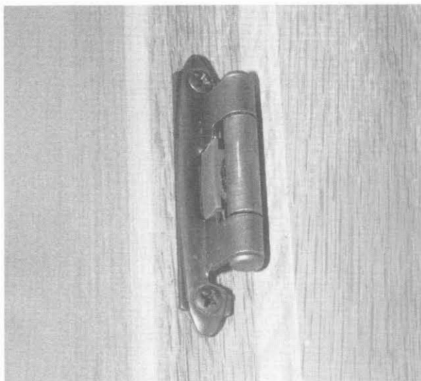
North American traditional hinges are simple to install on face-frame cabinets.
