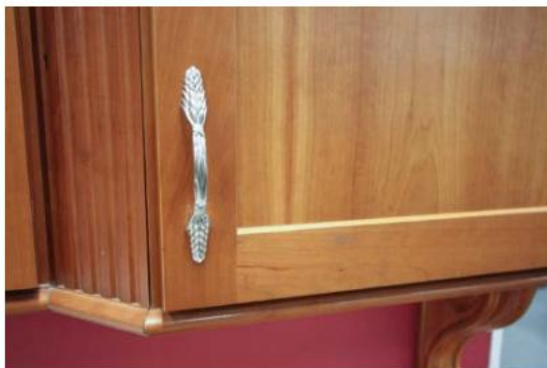
This door has a Shaker-style look, but it is modified with a chamfered inside edge, which makes it easier to keep clean.
