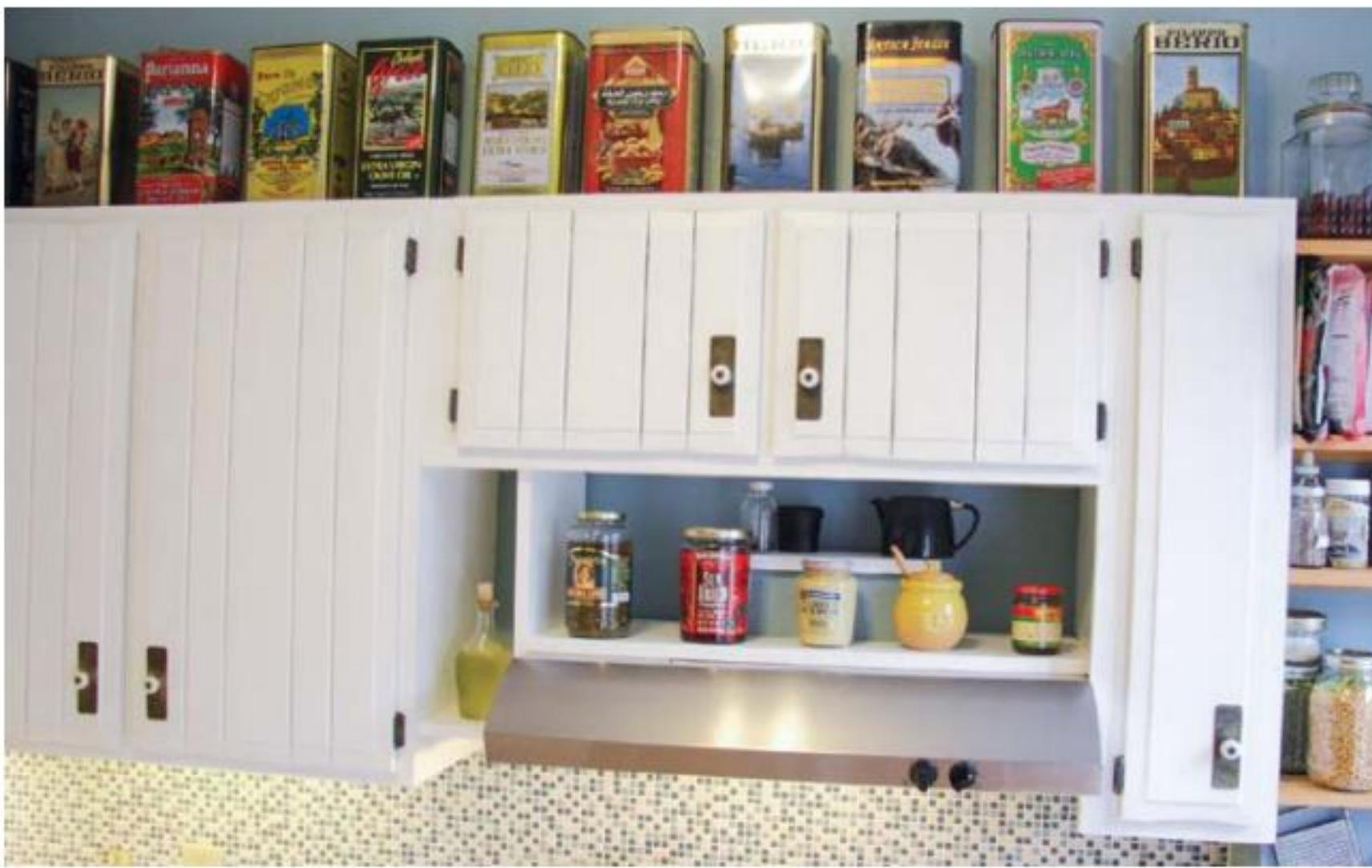
Cottage-style doors often use tongue-and-groove joinery. These doors are held together with cleats on the back.
