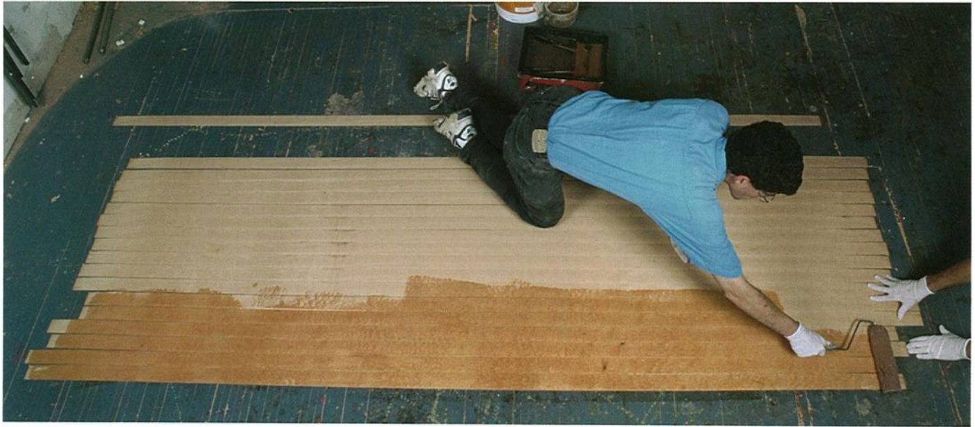
Photo C: There is a lot of surface area to cover with glue, so use a paint roller. The dried glue on the floor shows what happens if you don't use a tarp. I'd be more careful at home. (Photo by Strother Purdy, © The Taunton Press, Inc.)
