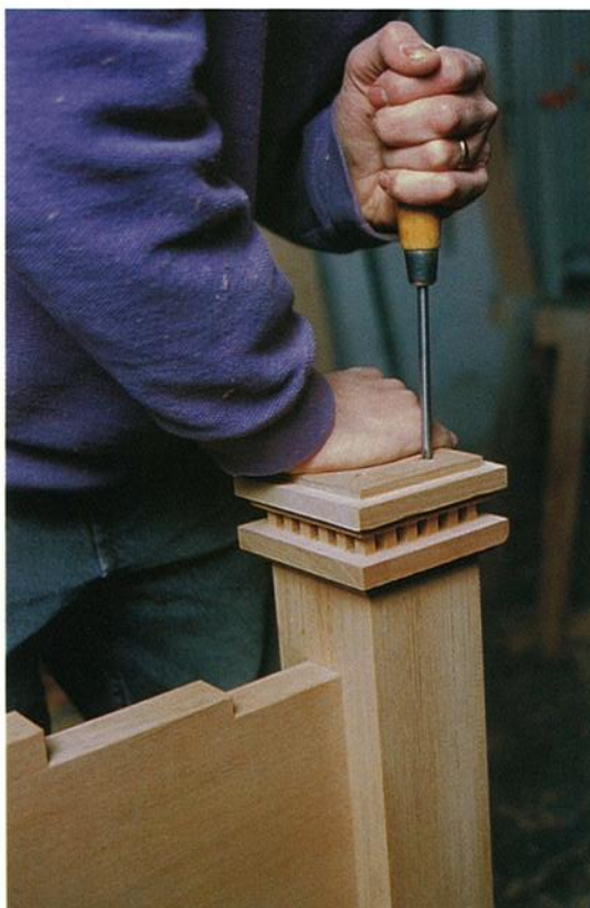
Photo J: Hold the capital carefully in place, then screw it down. Before you drive the second screw, be sure the capital hasn't shifted.
