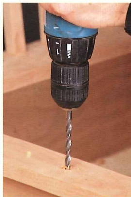
Now drill a hole (either 3/8" or 1/4" in diameter) that's about 3/8" deep.
