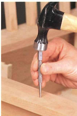
If there's a nail in the location of the plug, set it as deeply as you can.
