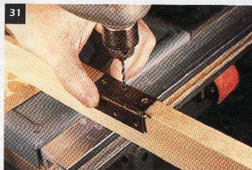
31. Hinges should fit snugly into the mortises and, as you're dealing with a very hard material, it's best to drill pilot holes before applying the screws.
